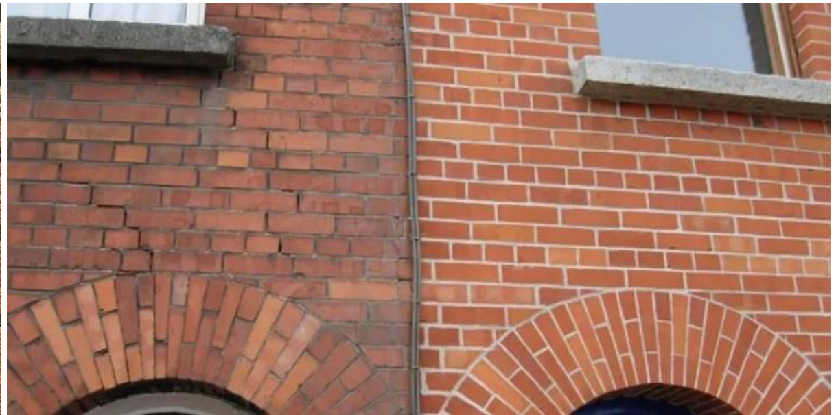
Example of masonry wall with a similar look that has been improved in appearance through repointing works
