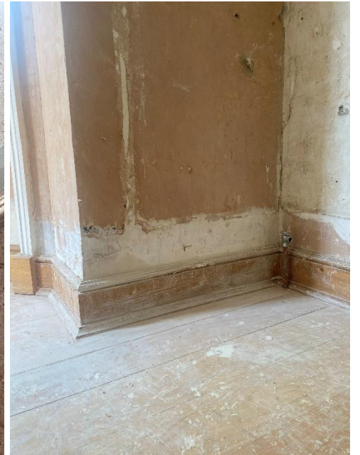
Ground Floor Section of the Original Skirting Removed
