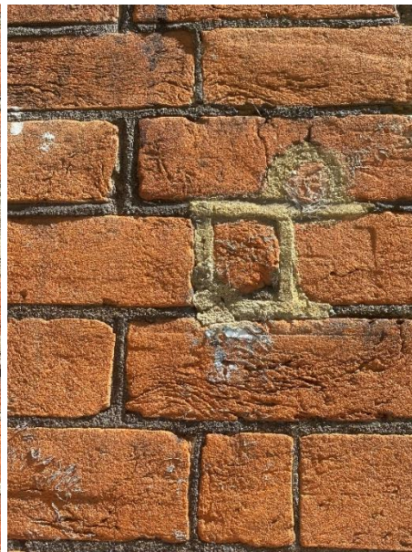
Site Photographs of the masonry wall with different mortar
