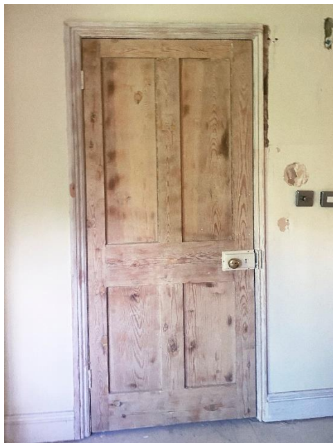
Internal Four-Panelled Doors
