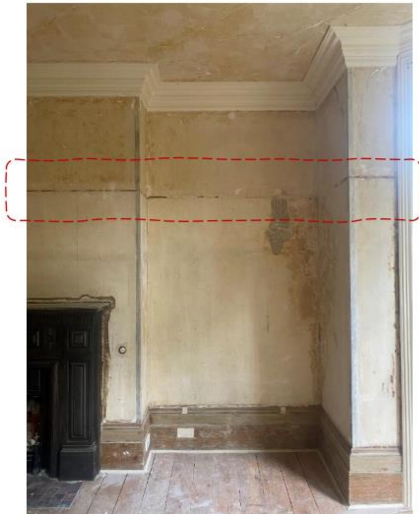
Evidence of existing picture rails to be reinstated throughout the building in existing locations
