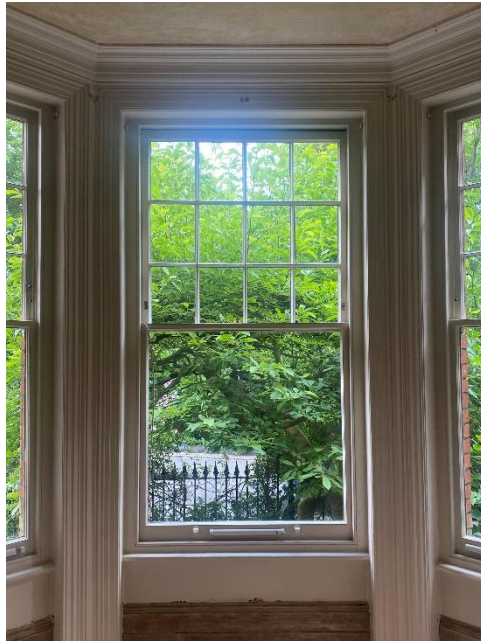
Single Glazed Timber Sash Windows With
