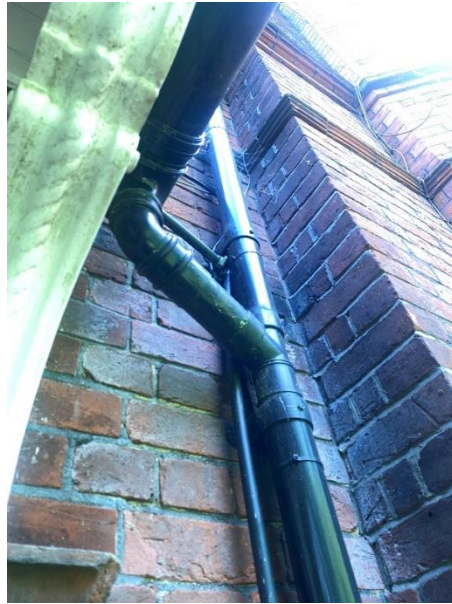
Site Photographs of the existing black uPVC Soil Vent Pipes
