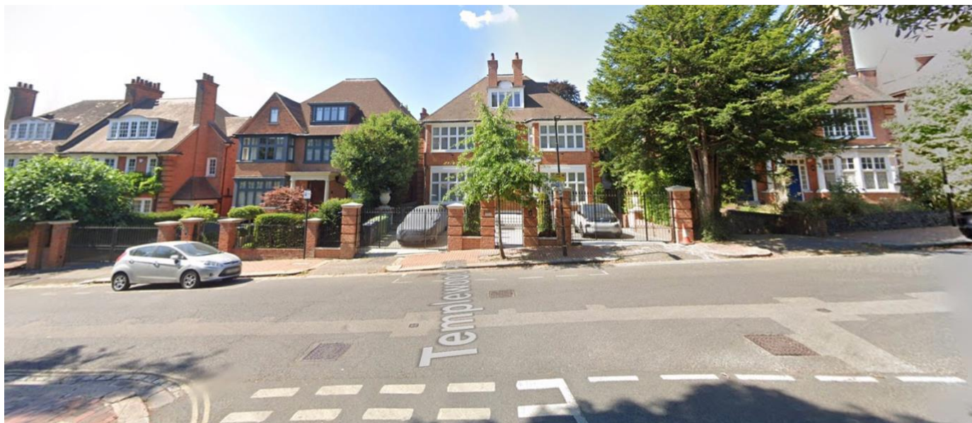
Figure 3: Photo of 59 Redington Road, with 57 to the left and 61 Redington to the right of the image.
