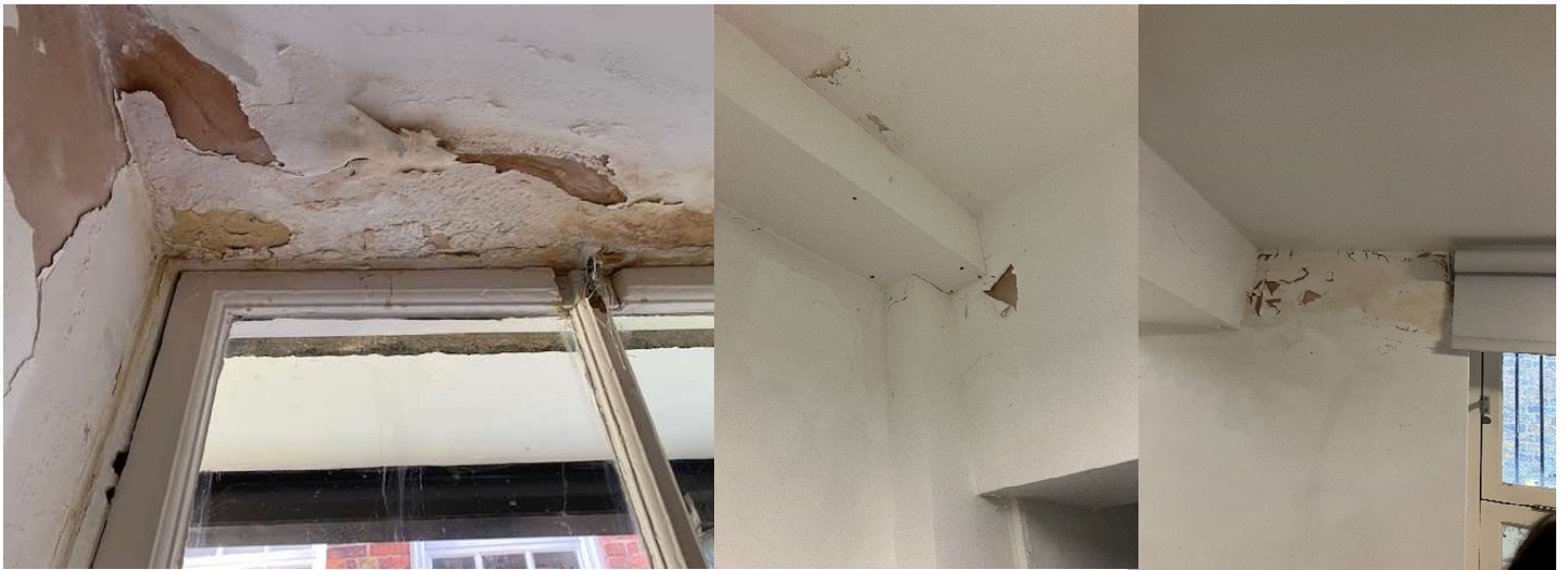
Figure 4: Photographs of internal damage.
