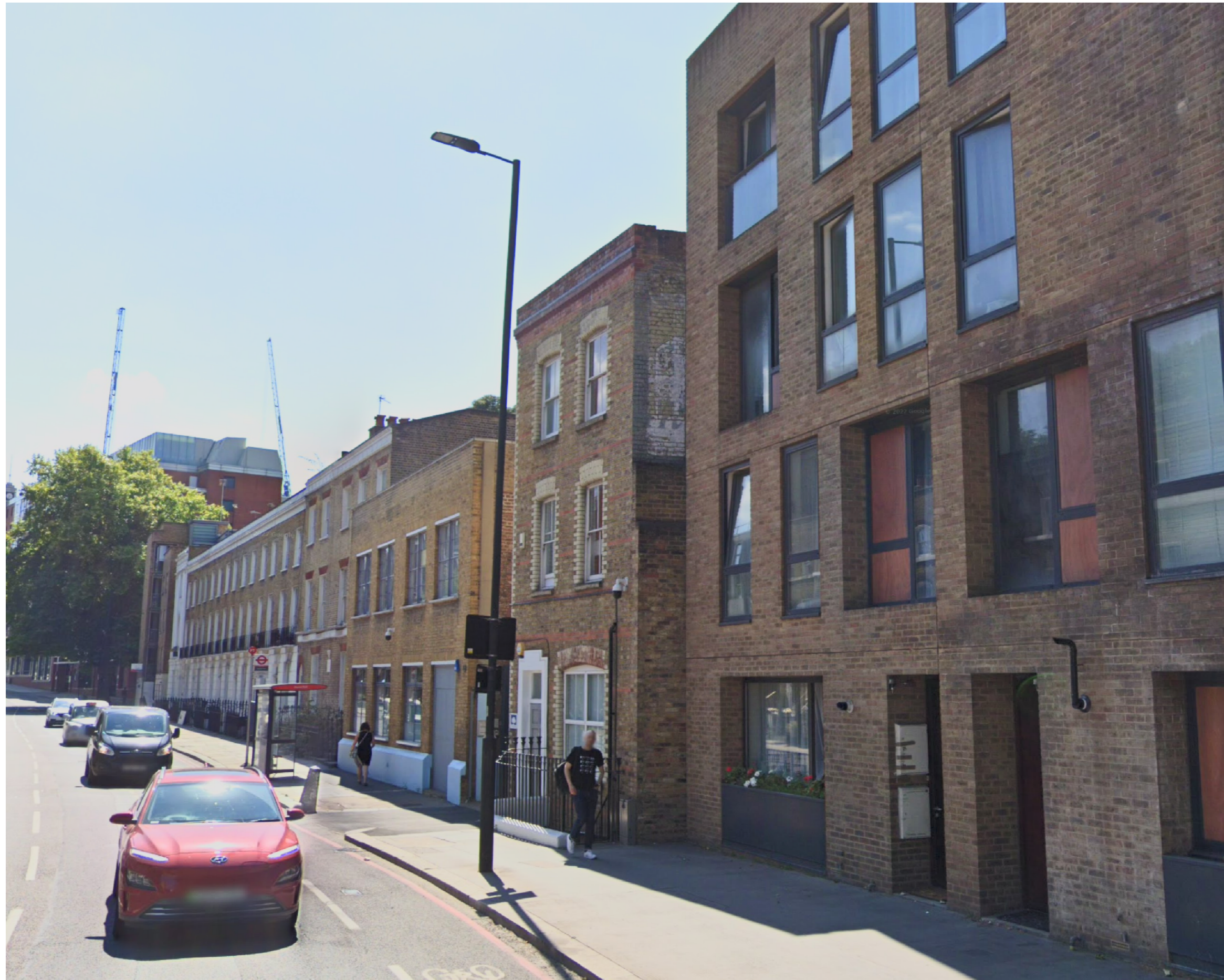
EVIDENCE OF No.71 ON PARTY WALL OF No.69
