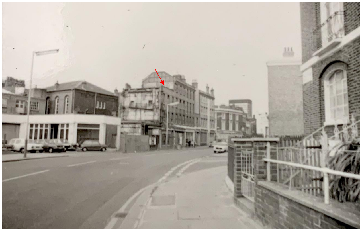
Fig 2: A c. 1978 photo of King's Cross Road, looking north, with the red arrow showing the Victorian building that predated the present 93-95 King's Cross Road. © Camden Archives
