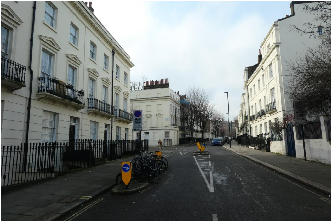
Photo 6: The listed terrace at 1-7 Frederick Street.
