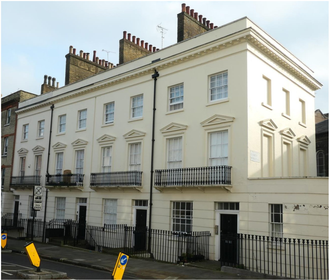
Photo 5: The listed terrace at 1-7 Frederick Street.
