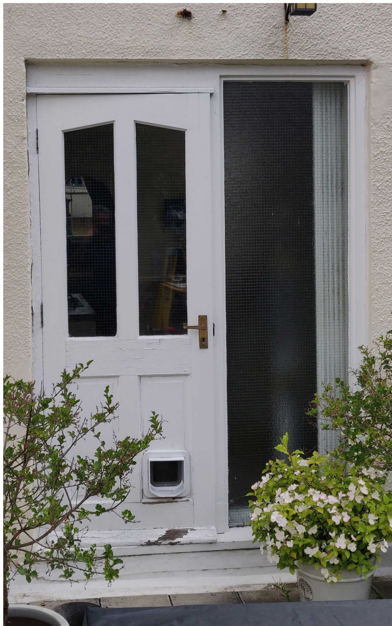
1 Existing Unsympathetic Timber Door & UPVC Window
