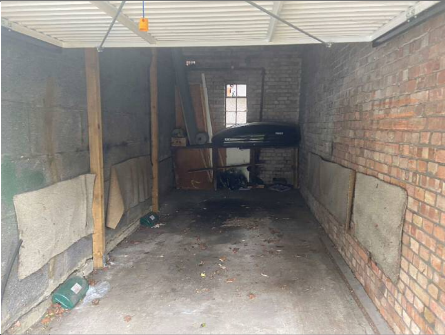
Photo 5: Internal photo of one of the garages.
