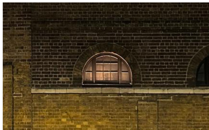
4 (Photos 4-8) Adjusted to 12.5% brightness. Photos and mock up were reviewed by TRACT on the 27th September 2023. We have received a positive collective feedback.
