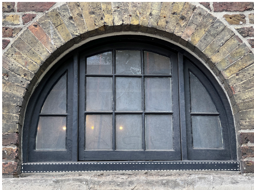
As existing window and frame. Proposed lighting will be mounted to the existing timber frame (indicated in dashed lines).
