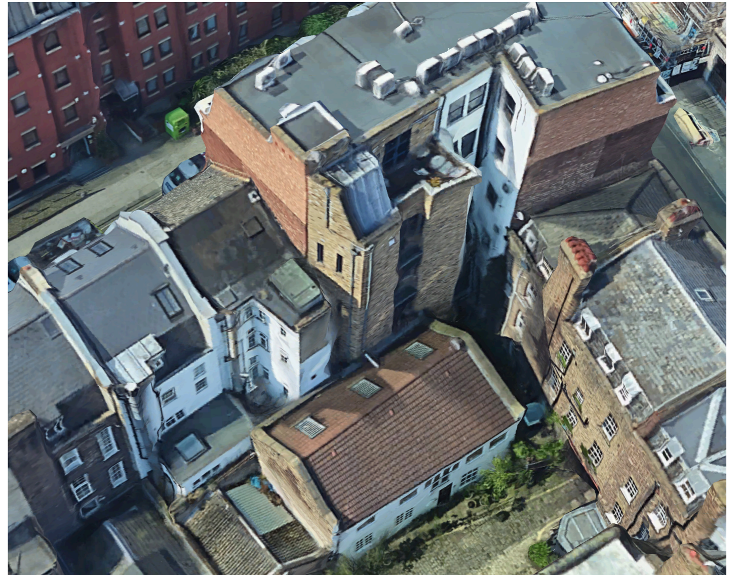
View showing blank walls to the rear of the property and AC units on the roof of the corner property
