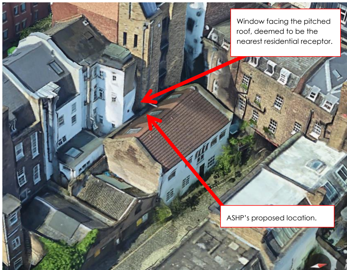
Figure 1 ASHP unit and nearest receptor locations
