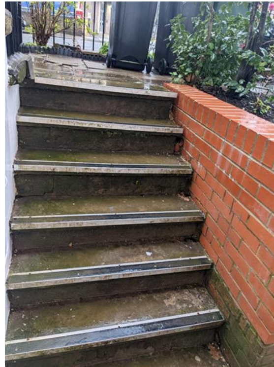
Existing stairs to lower ground floor entrance
