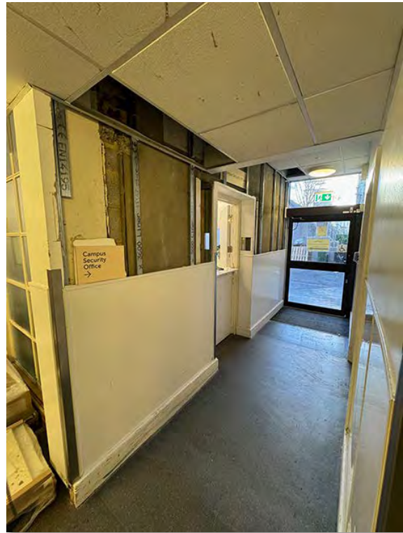
IMG_1458 lower ground entrance corridor – upper section drylining removed to assess structure
