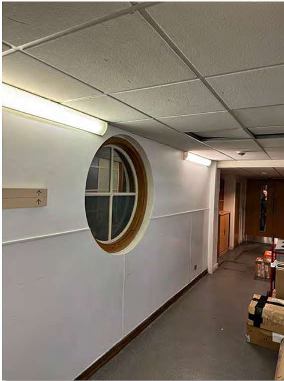
IMG_0921 later addition oak framed crittall window within interior corridor studwork
