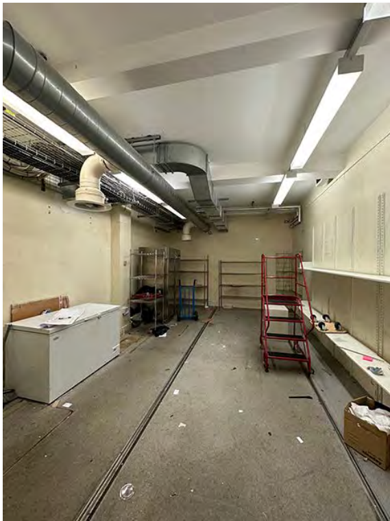
IMG_4735 area 0L/007 decommissioned kitchen dry store
