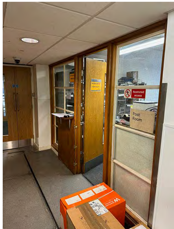
IMG_0900 later addition glazed crittall screen & oak framing
