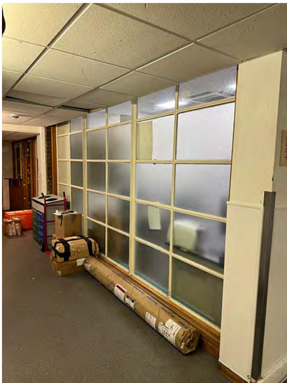
IMG_0919 later addition glazed crittall screen partition
