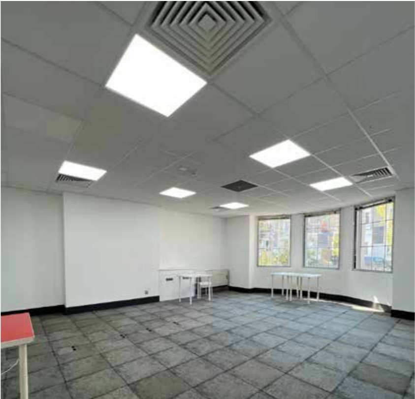
Figure 5.7 Existing Photograph showing suspended ceiling at ground floor level
