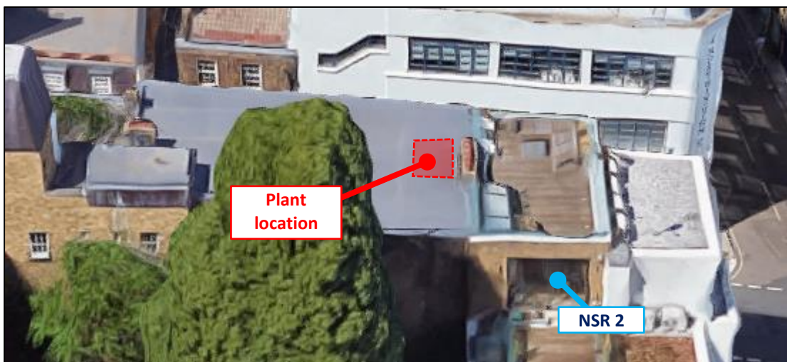
Figure 6.3 Noise sensitive receiver 2 and proposed plant installation location
