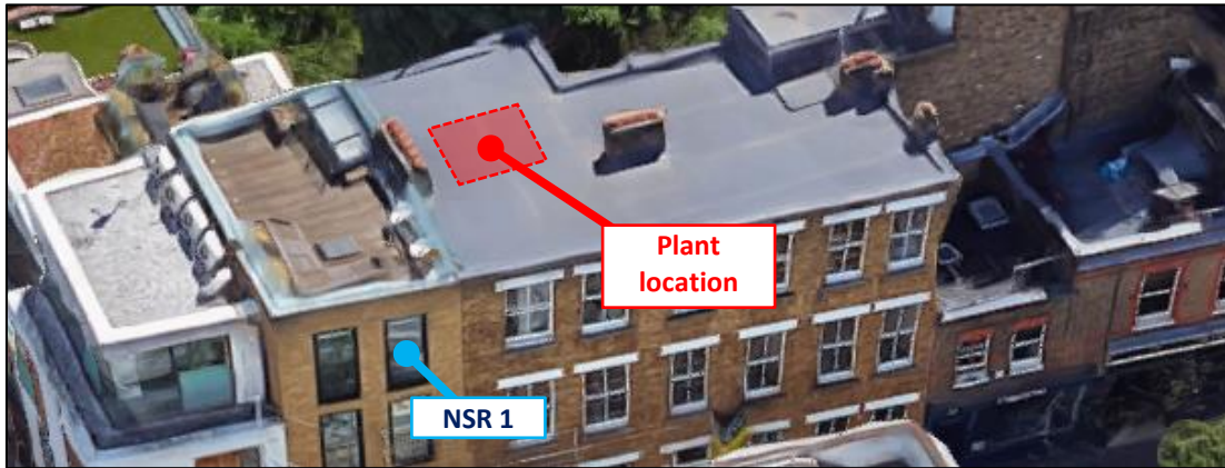
Figure 6.2 Noise sensitive receiver 1 and 9 proposed plant installation location
