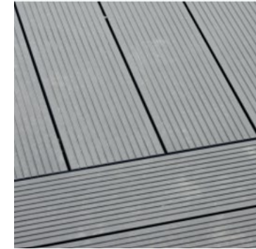
Fig. 3: Aluminium decking as per approved drawings
