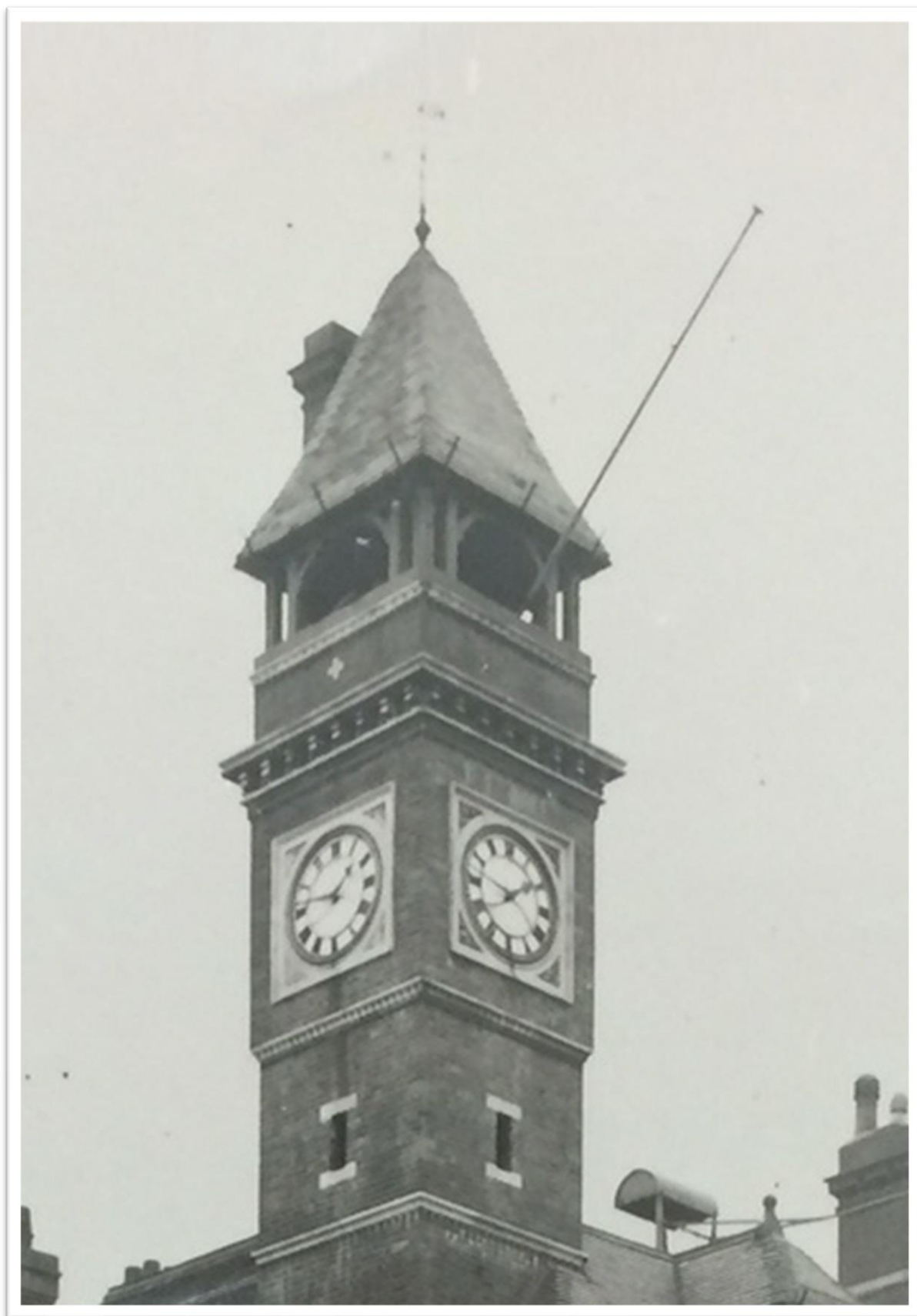
9. Detail of 1905 photograph, showing the tower roof with its finial and flagpole. Precautions are in place to prevent tiles falling to the ground
