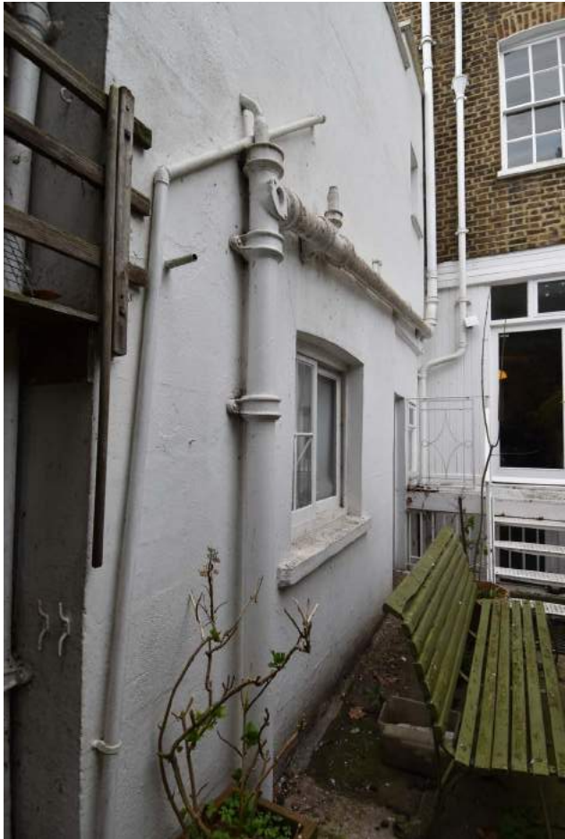
3.7 Return elevation of the closet wing extension (2023, Donald Insall)
