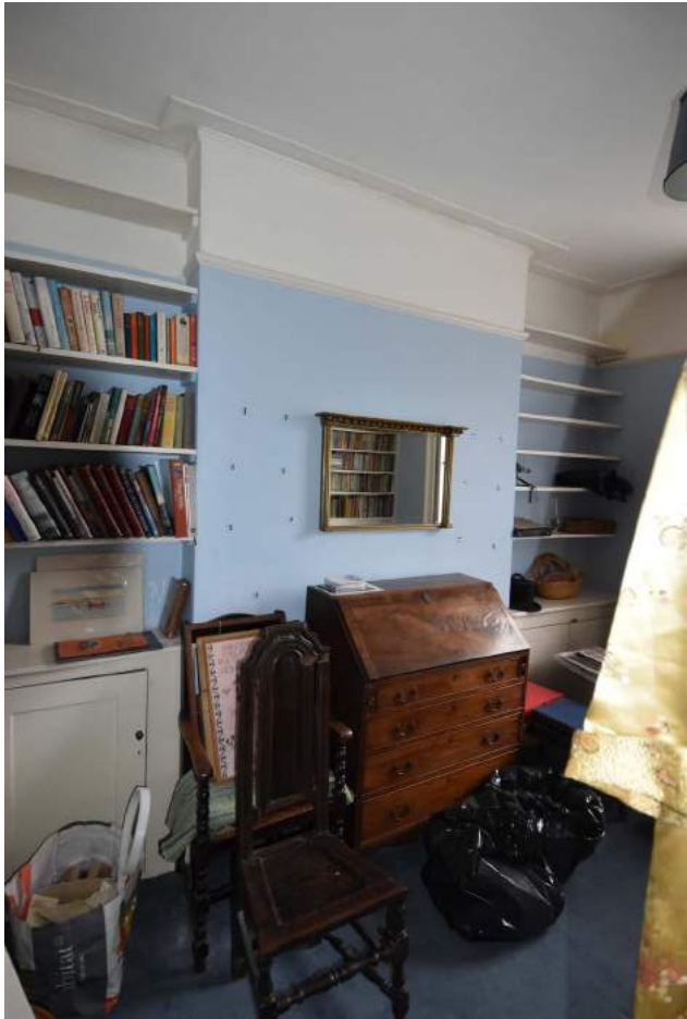
3.42 First floor rear room north wall in F3 (2023, Donald Insall)
