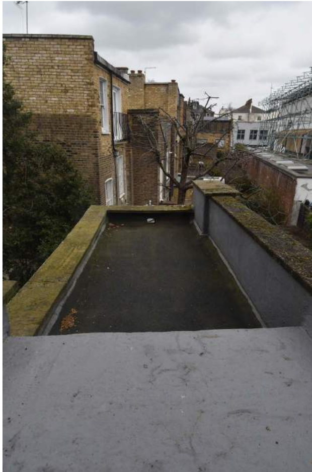
3.8 Modern flat roof to the closet wing extension (2023, Donald Insall)
