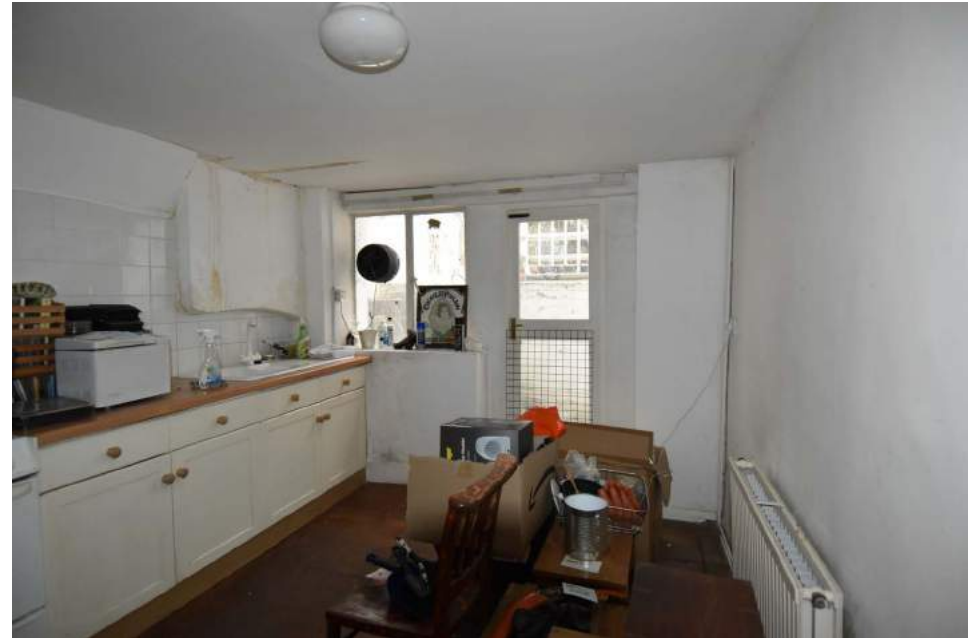
3.18 Utility kitchen east wall in room LG2 (2023, Donald Insall)
