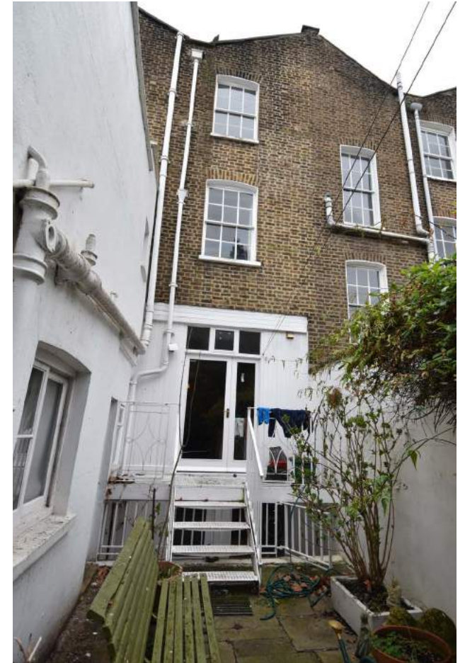
3.3 Rear elevation showing the rebuilt ground floor (2023, Donald Insall)
