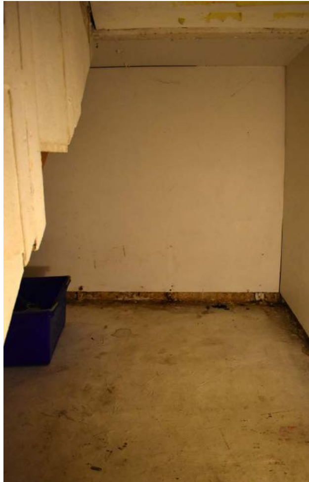
3.16 Interior of under-stairs cupboard (2023, Donald Insall)
