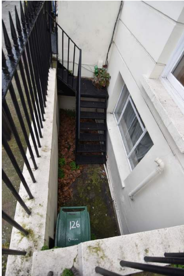
3.2 Front lightwell showing the modern replacement stair (2023, Donald Insall)
