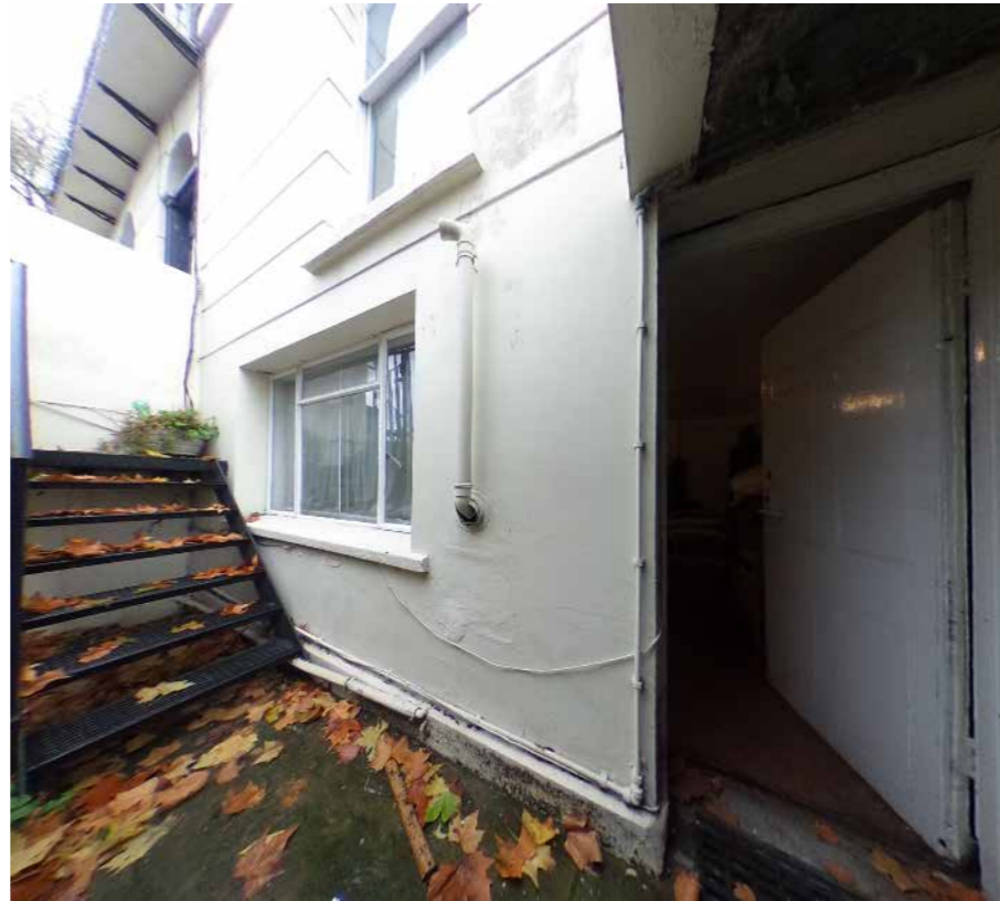
Lower Ground Floor entrance
