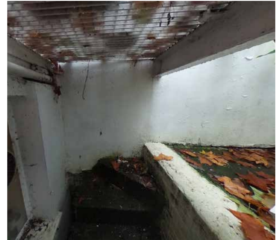
Lower Ground Floor garden access
