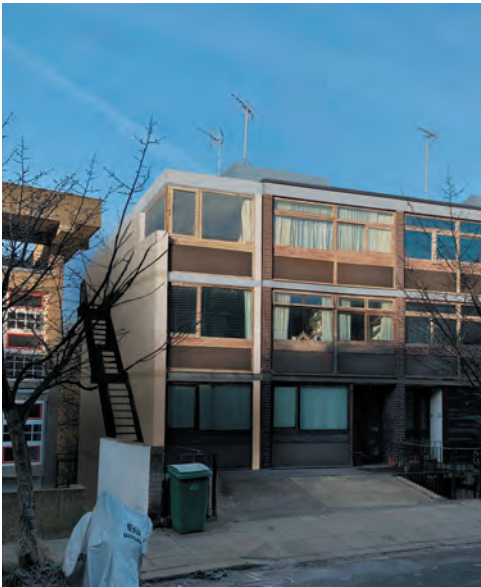
Rendered view of no. 80 extension and externally insulated flank wall
