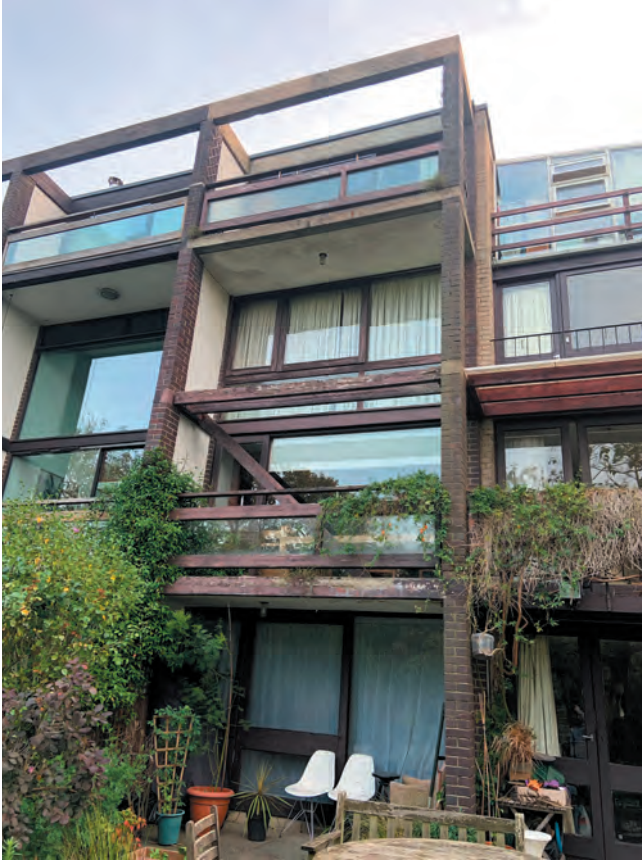
Existing rear view photos of South Hill Park
