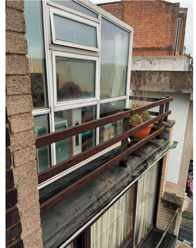
Existing rear view photos of South Hill Park unsympathetic additions of balustrades, greenhouse and glazing details
