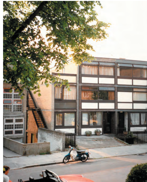
Views of the of the terrace in 1970-80s showing that the concrete ring beams appear to have been painted and some glazing has been replaced. A First Floor extension has also been introduced to no.80 designed by Gill Howell with a second Floor terrace
