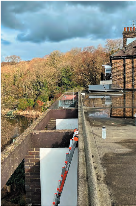
Existing roof towards rear garden
