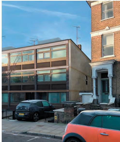
Rendered view of flank wall with external insulation at no90 end of terrace
