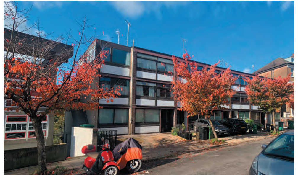
View of the terrace at present showing now dark, aluminium framed windows and the concrete ring beams painted to a darker colour than the previous iterations. Additions to the no.80 extension were made on the second floor with a lean-to bedroom and greenhouse added, compromising the overall design consistency.
