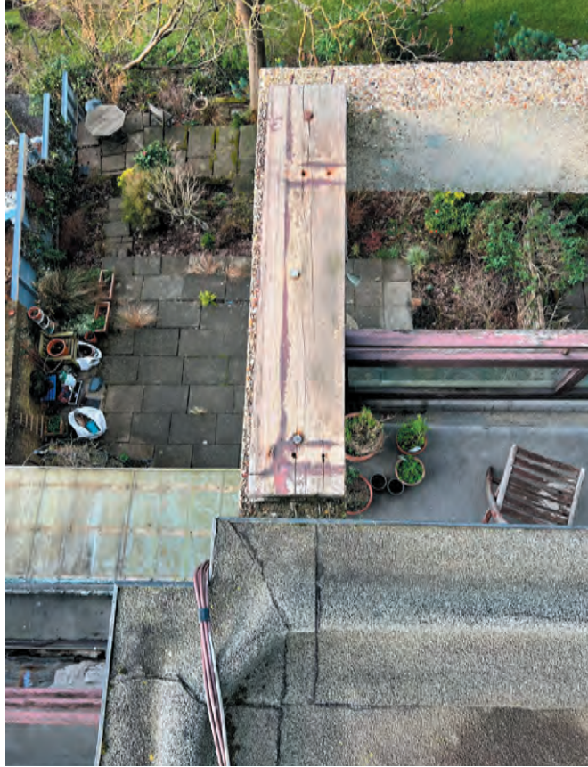
Existing rear view photos of South Hill Park showing rotten timber capping plates over the rear concrete terrace frames
