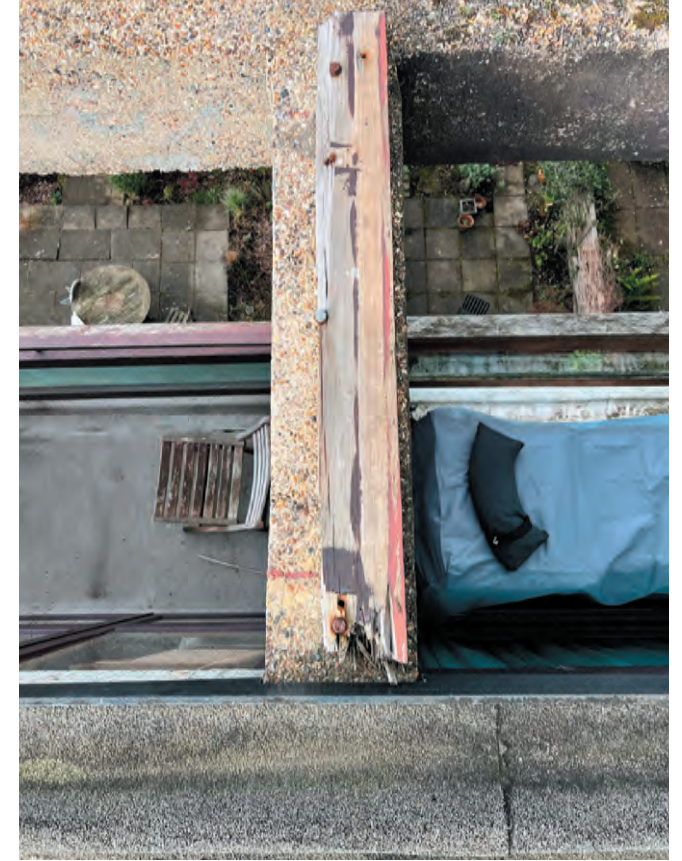
Existing rear view photos of South Hill Park showing rotten timber capping plates over the rear concrete terrace frames
