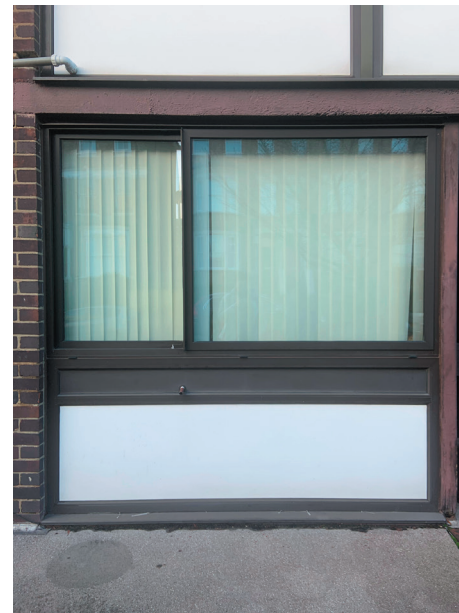
View of the Aluminium glazing at front
