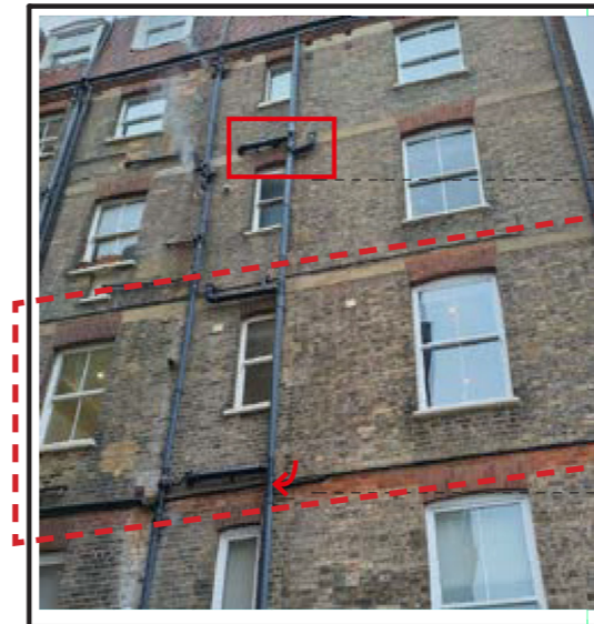
Location of new penetration through wall and exterior pipework (minor bend to existing soil pipe) to match existing two floors up as per 10_Existing Proposed Plans-Photo C
