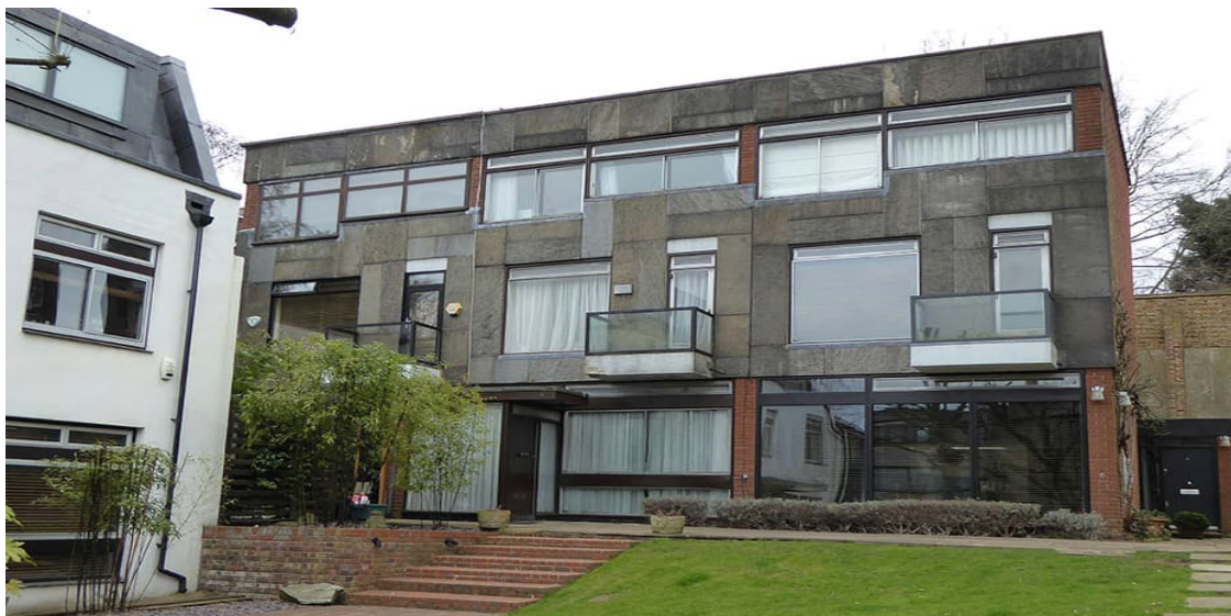
Figure 2- Front Elevation Terrace 4,5,6 – (1,2,3 to the left in picture)
