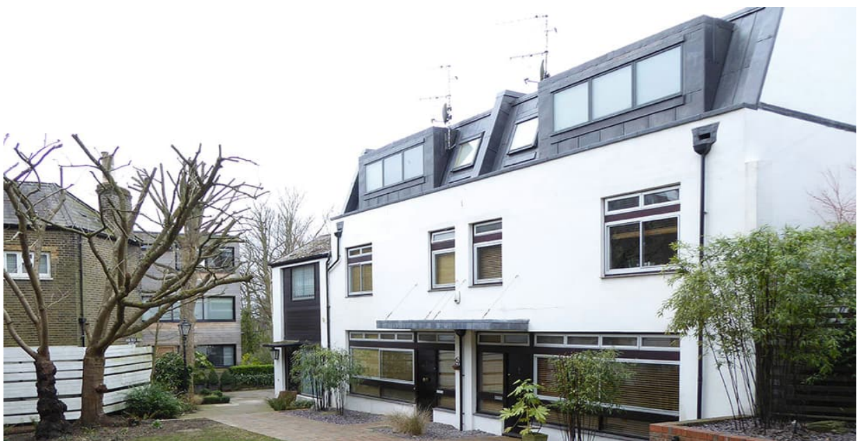
Figure 3- Front Elevation Terrace 1,2,3 – (All windows are a recent replacement)
