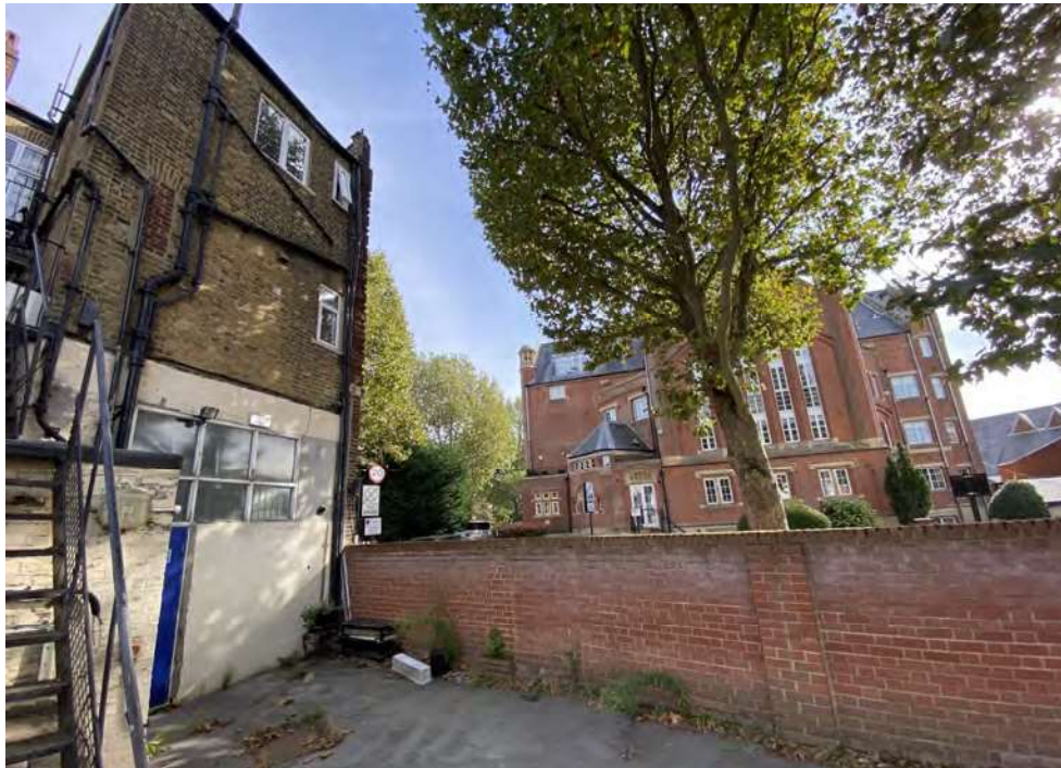
Photographic plate showing T2 in proximity to the rear of number 529. (ROAVR, 2023)
