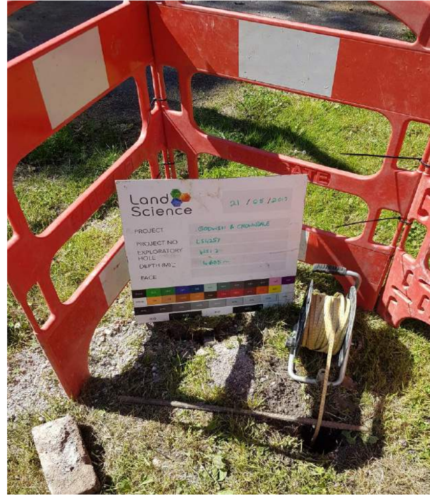
WS1.2 Soakage Test
