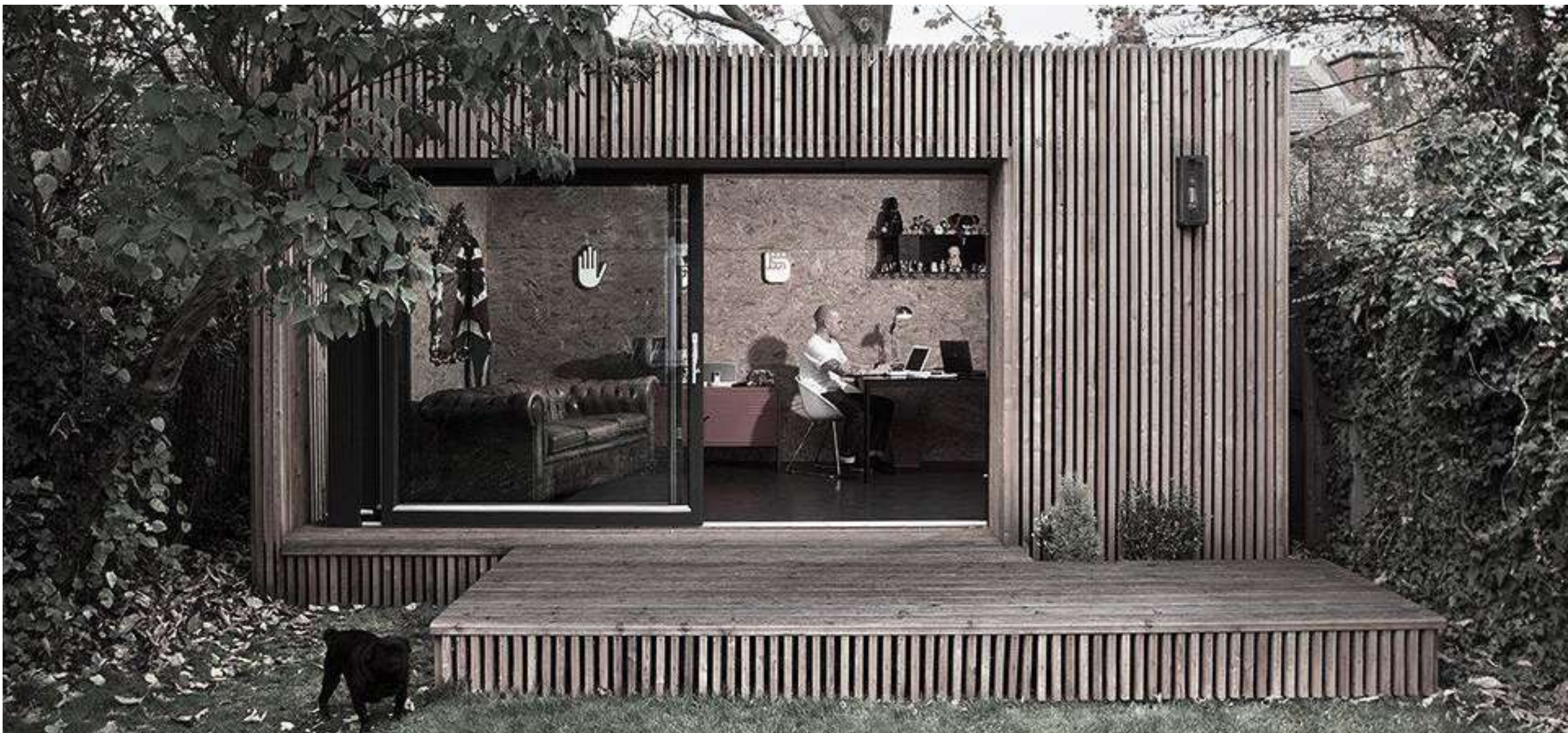
Image 01 - Example of flat top / box form & vertical timber cladding
