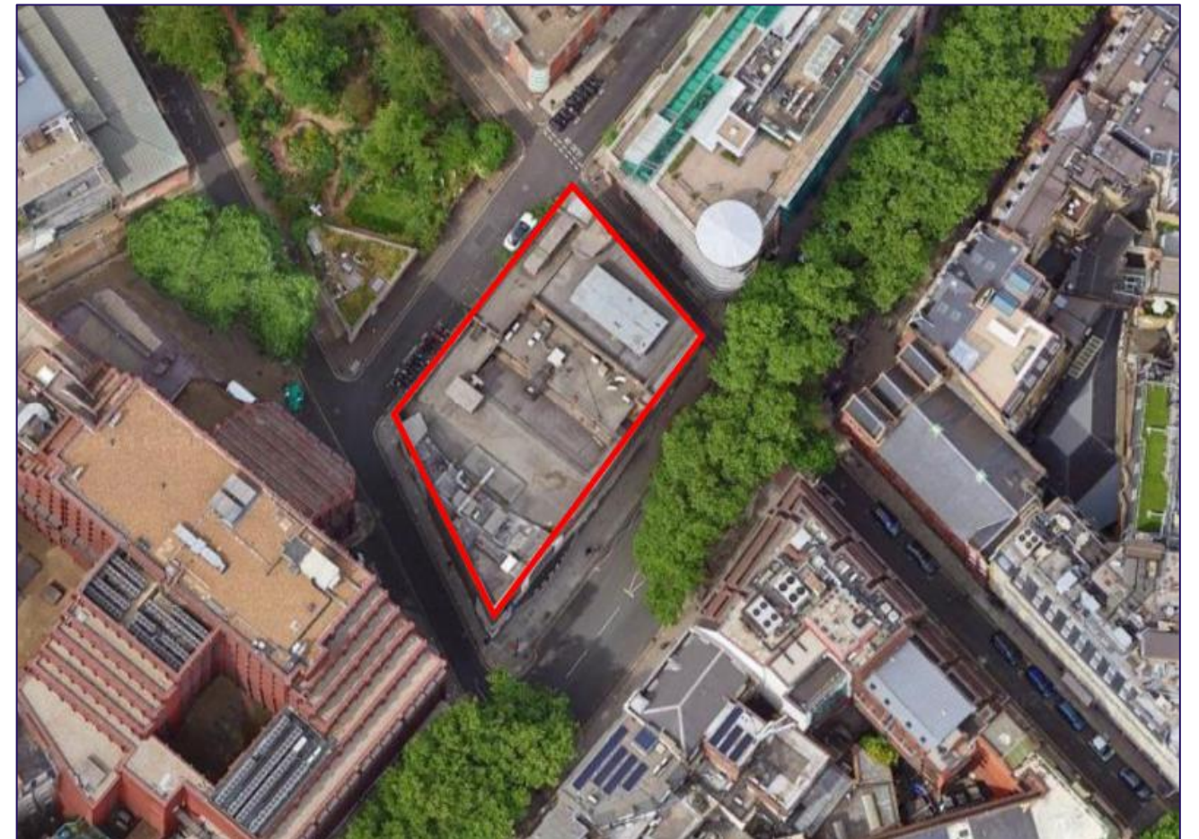
Figure 2—2 View of Saville theatre from above (Courtesy – Google Maps)
