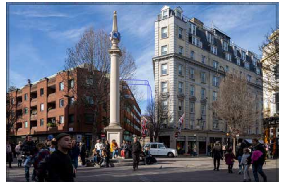
Figure 9.3 Verified view of the Proposed Development looking north on Mercer Street from Seven Dials
