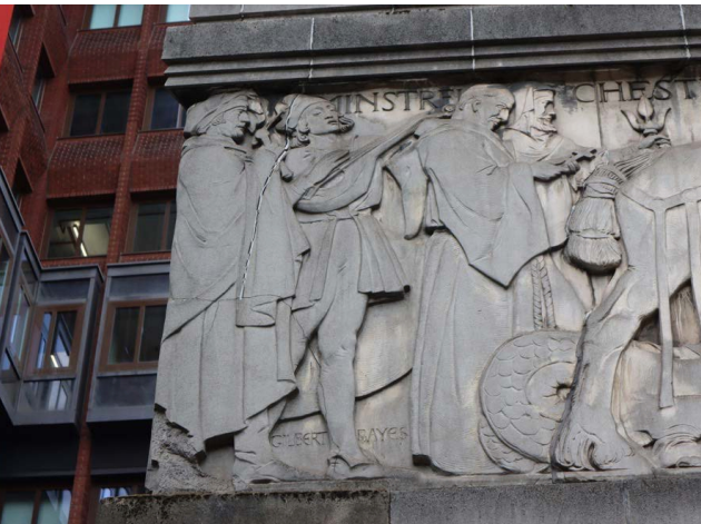
F - GILBERT BAYES FRIEZE CRACKING THROUGH THE MORTAR JOINTS AND PRE-CAST ARTIFICIAL STONE
