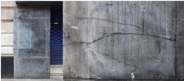
B - MAIN ENTRANCE MARBLE CLADDING IN POOR CONDITION
