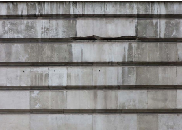
G - FINE CRACKING AND SPALLING IN RUSTICATED PORTLAND STONE, POTENTIAL LAMINAR CORROSION IN EMBEDDED STEEL WORK
