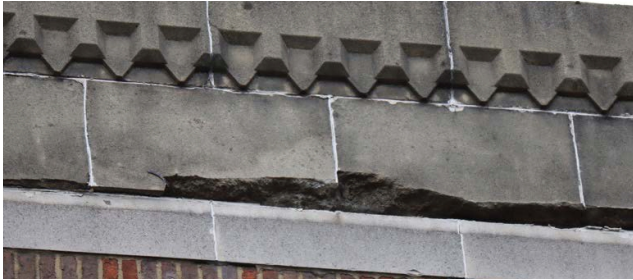
H - CRACKING AND SPALLING IN ARTIFICIAL STONE PARAPET, LIFTING AND DISPLACEMENT OF STONE BLOCKS, PROBABLE LAMINAR CORROSION OF STEEL STRUCTURE
