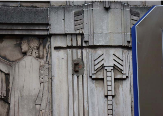
E - CHASE CUT INTO THE CAST STONE WINDOW SURROUND, CORRODING STEEL CHANNEL IS PRESENT
