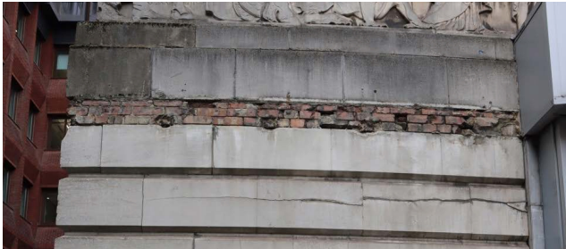
C - CRACKING IN THE RUSTICATED PORTLAND STONE
