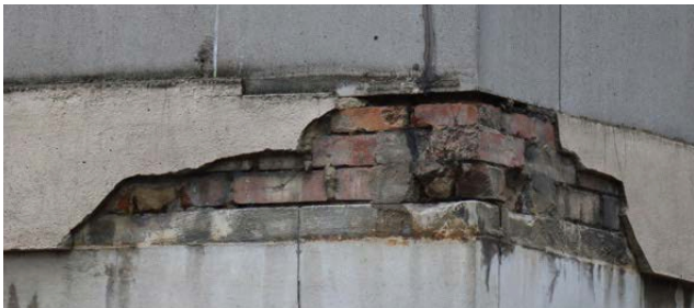
A - FELTON BRICK BAND PARTIALLY RENDERED WITH VERTICAL CRACK PASSING THROUGH STONE AND BRICKWORK
