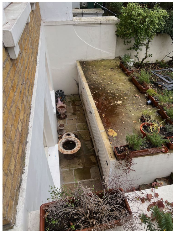
fig 1.4 View of concrete store cupboards to front well
