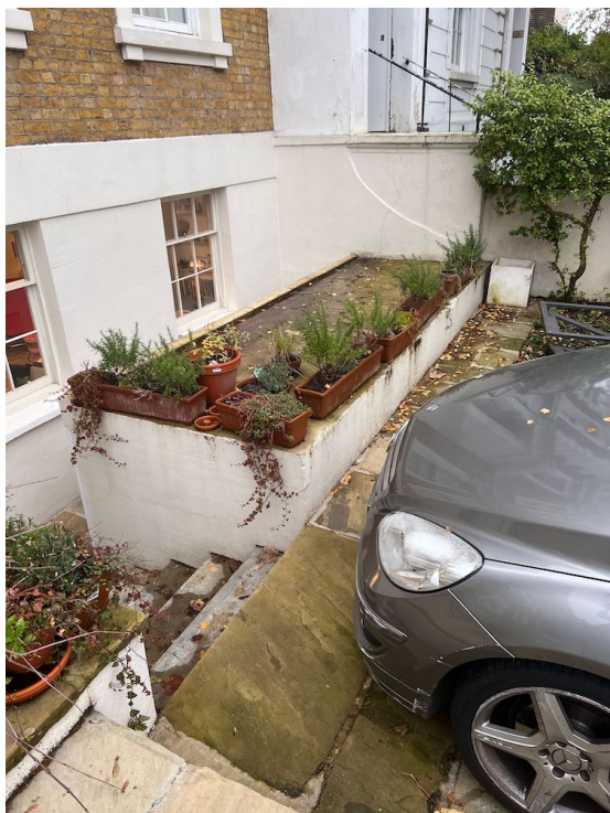
fig 1.3 View of concrete store cupboards to front well
