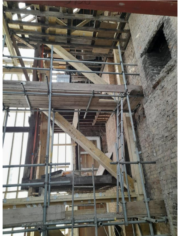
Figure 2 - Right hand side of Braced Frame
