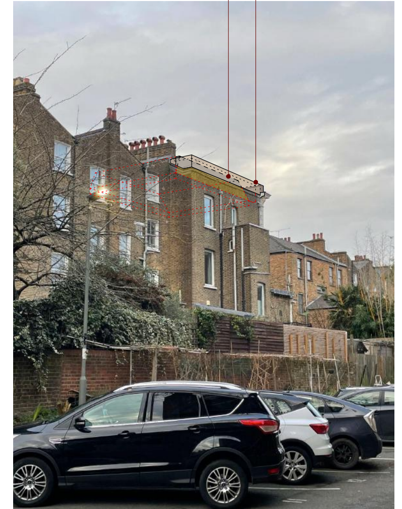
C VIEW FROM WILLINGHAM TERRACE - LOOKING TOWARDS THE REAR OF 66 FALKLAND ROAD
