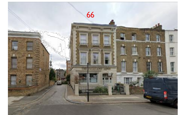
E VIEW OF 66 FALKLAND RD - LOOKING TO WILLINGHAM TERRACE
