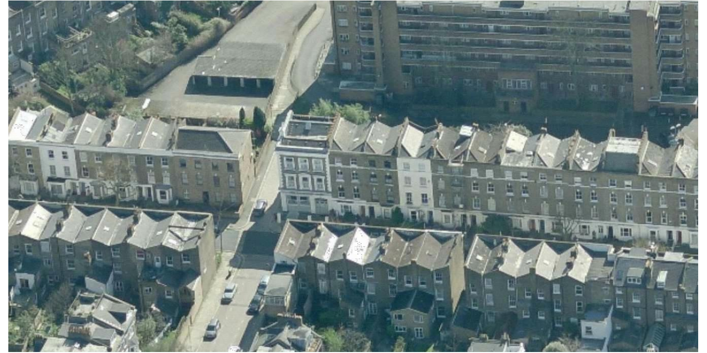
B AERIAL VIEW FROM THE NORTH
