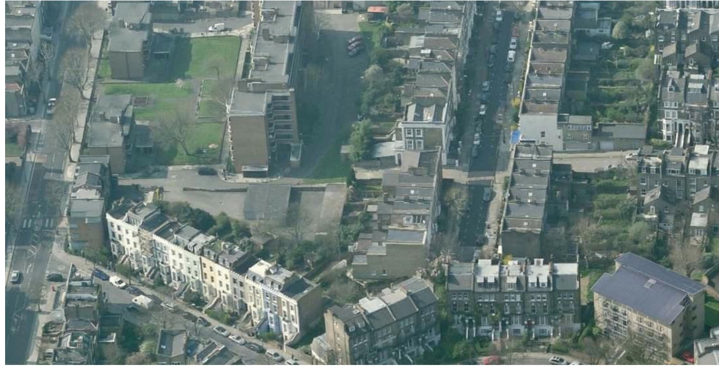
A AERIAL VIEW FROM THE WEST
