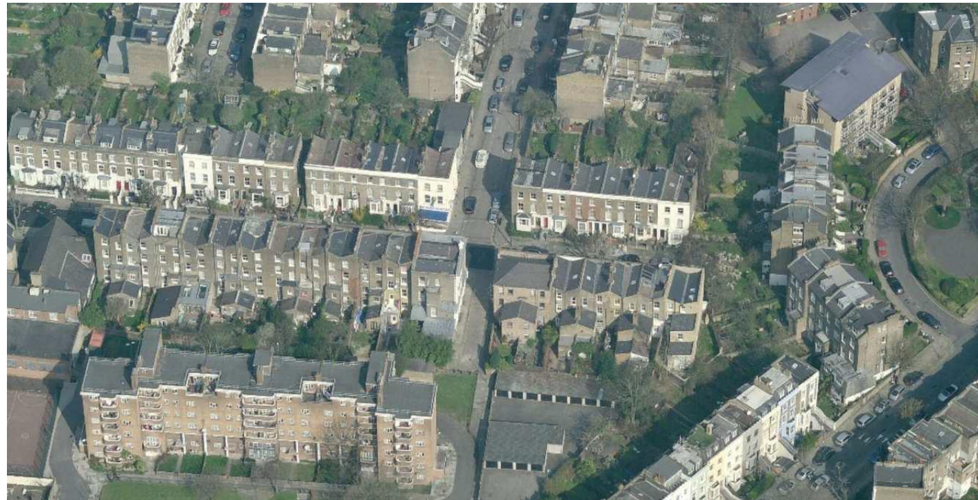
C AERIAL VIEW FROM THE SOUTH
