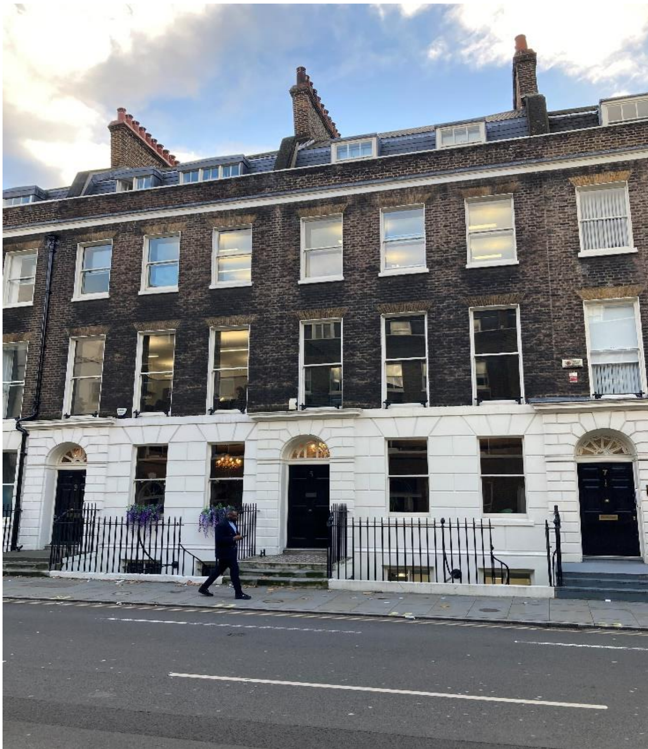
Figure 3.2 – Exterior of 3 and 5 Gower Street.
