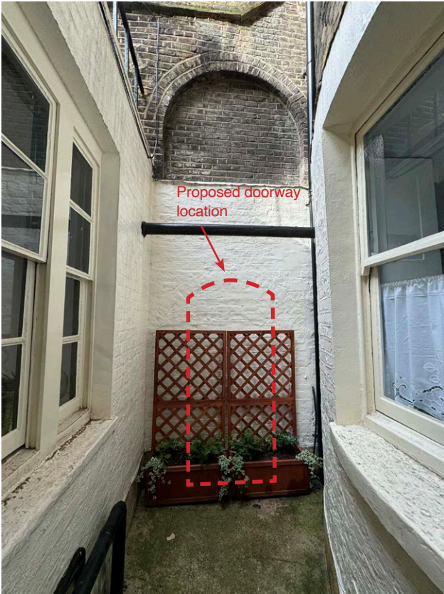
No. 3 lightwell looking towards no. 5 party wall
