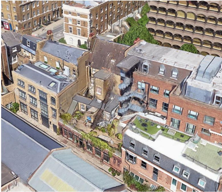
Figure 2.2 Rear View of the Site in Comparison with Adjoining Buildings
