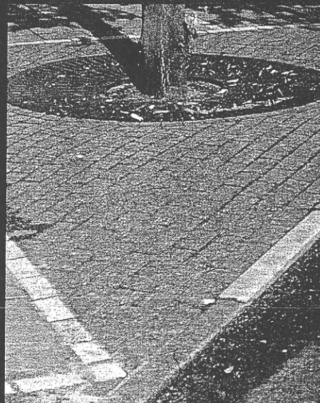
Brick pavers allow good air exchange
