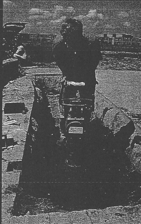
A whacker is used to compact the tree soil
