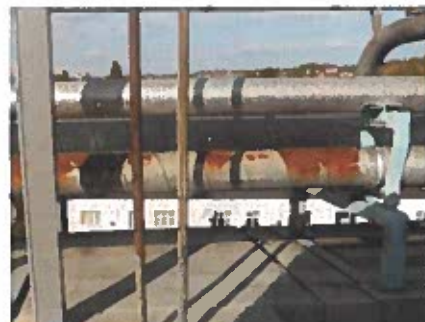
Roof structure located on Block A roof
