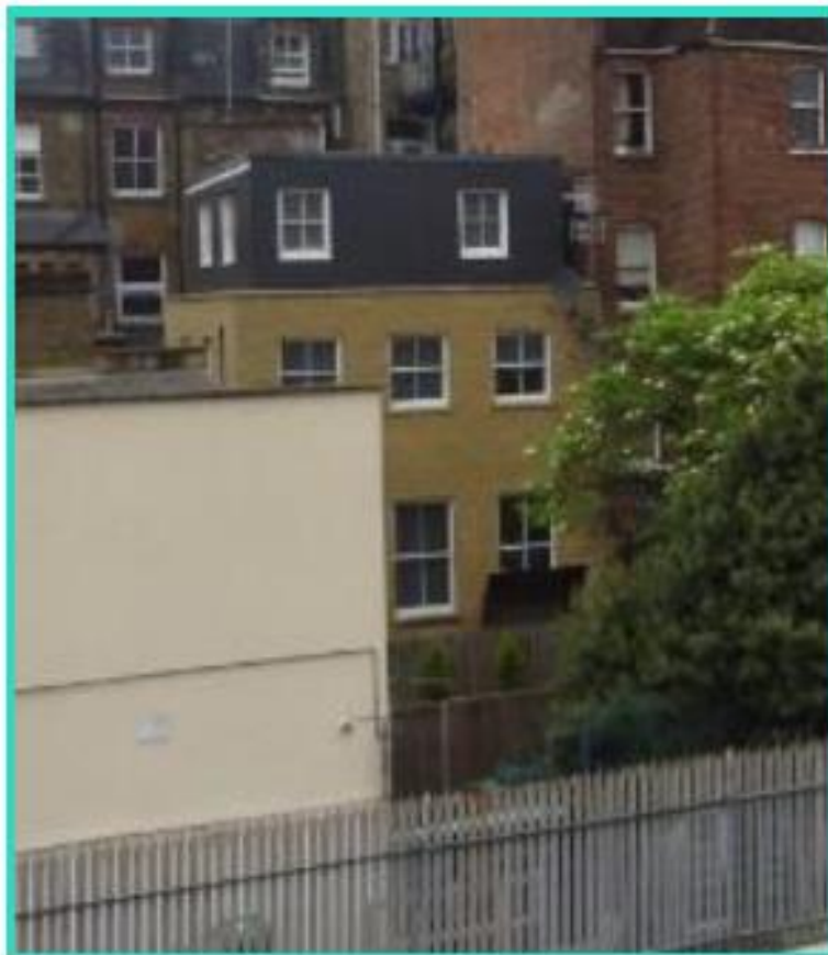
Figure 16 – Rear of 3 Blackburn Road
