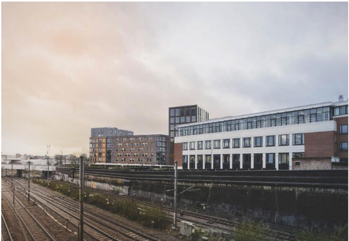
Figure: 11 – Proposed view looking east along the railway cutting from the bridge on West End Lane
