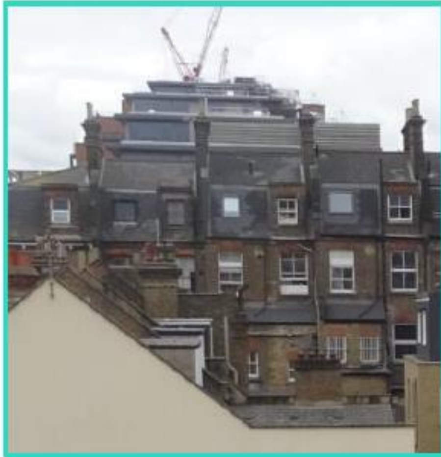
Figure 17 – 128-130 West End Lane
