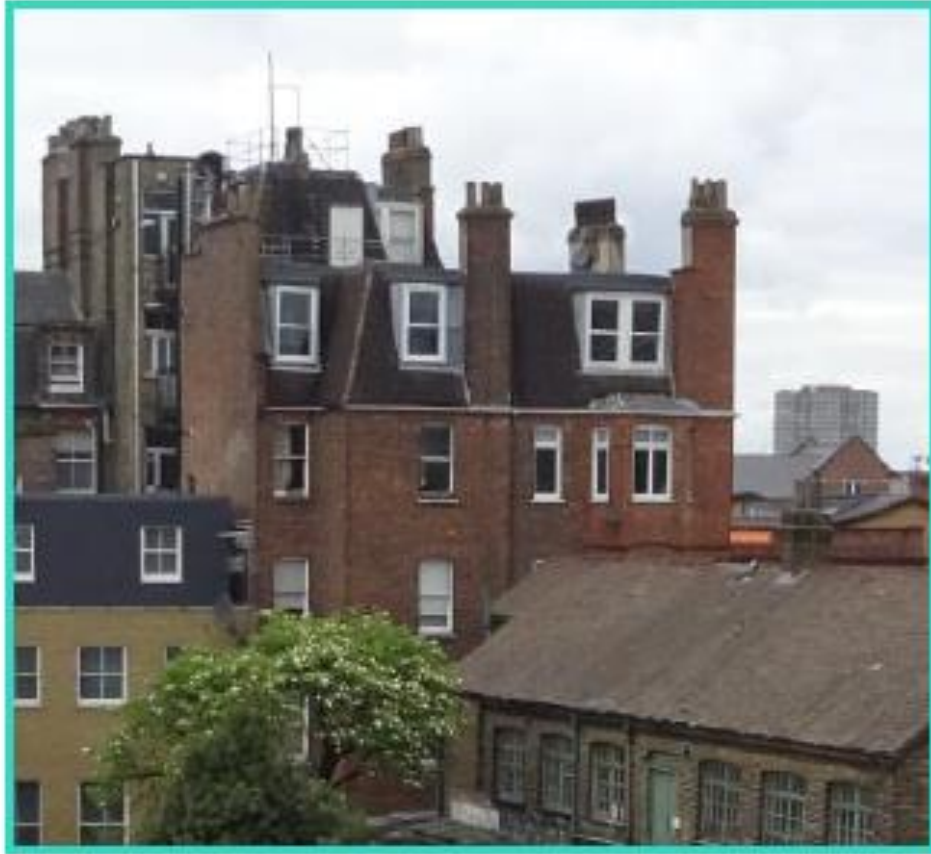
Figure 18 – 134-136 West End Lane
