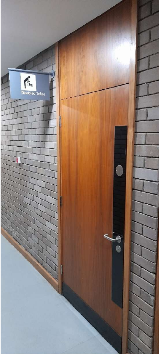
3: Existing DDA WC door – new CPT room door to match this as closely as possible
