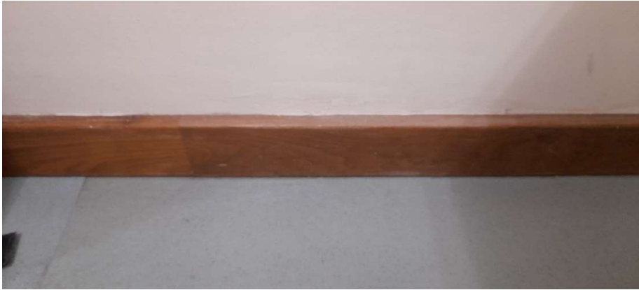
7: Typical Interview room skirting to be removed
