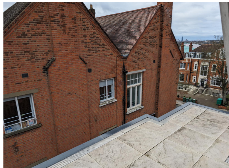
Existing flat roof viewed from Flat 7
