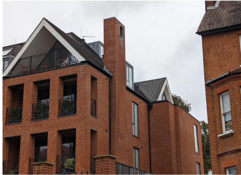
View from Netherhall Gardens showing existing flat roof to South elevation
