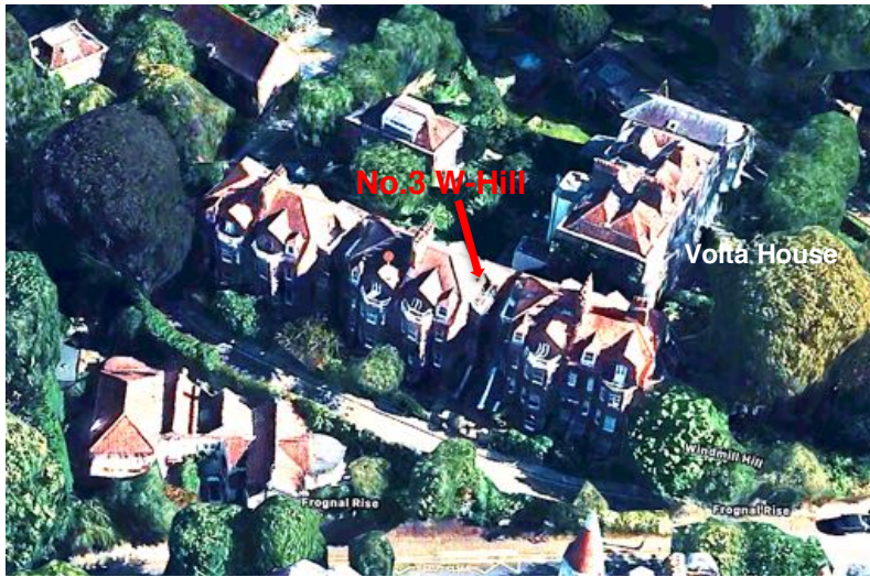
Aerial view from west (front) [from Google maps]
