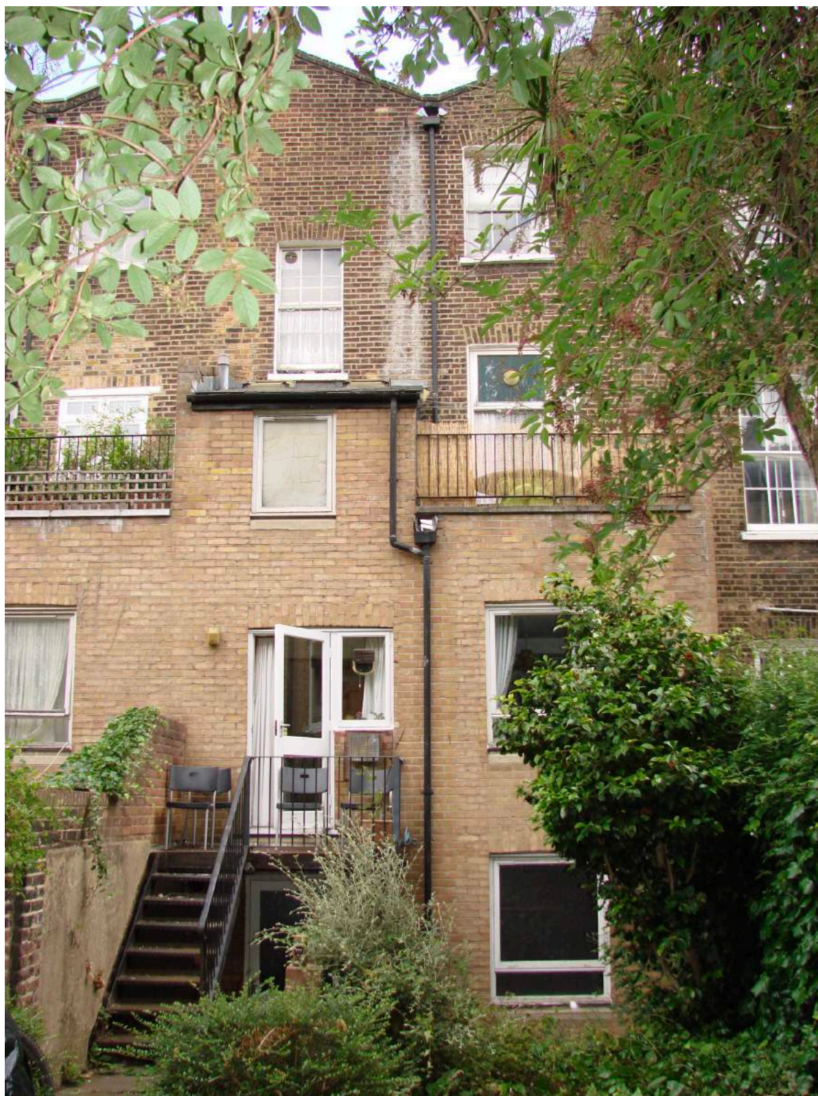
The Rear Elevation of No. 57. Inappropriate modern extension - No Heritage Significance. Surviving original sliding sash windows - Medium Heritage Significance. Overall - Low Heritage Significance.
