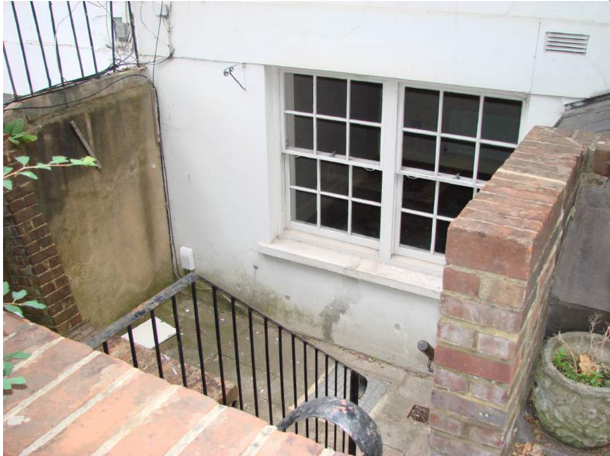
The basement floor elevation of No. 57. Modern altered window opening with paired sashes - Negligible Heritage Significance. Inappropriate modern alterations to the steps - No Heritage Significance. Overall - Low Heritage Significance.
