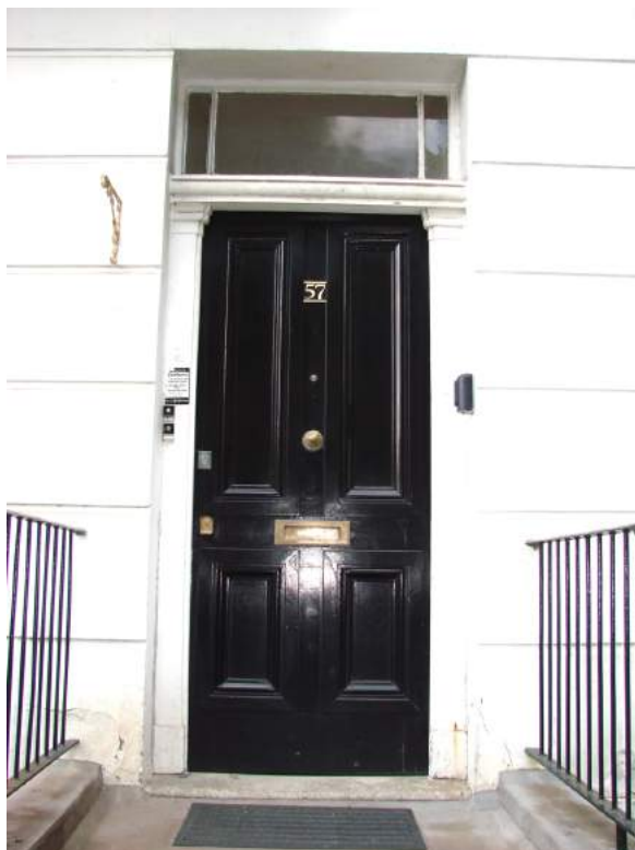
The Front Door. Original - High Heritage Significance. Inappropriate modern railings to sides - No Heritage Significance.
