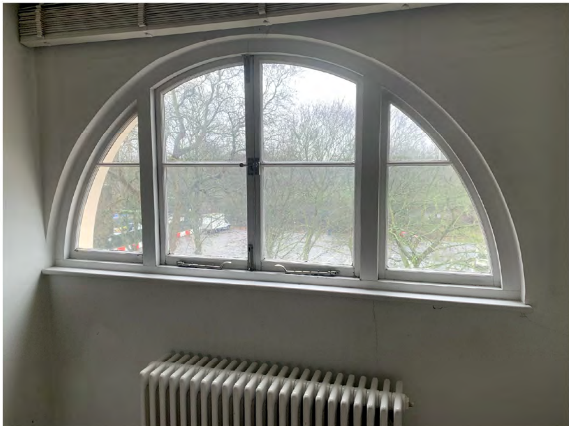
Plate 14: Oriel window to second floor
