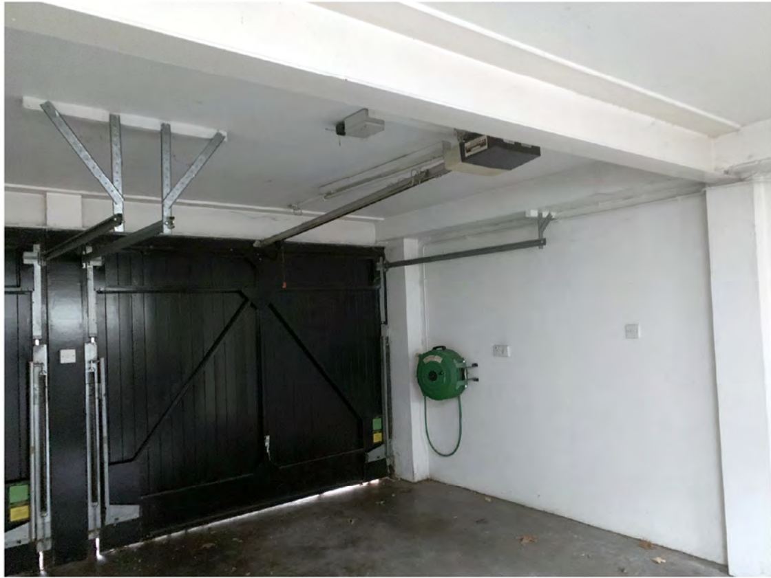
Plate 21: Interior to garage
