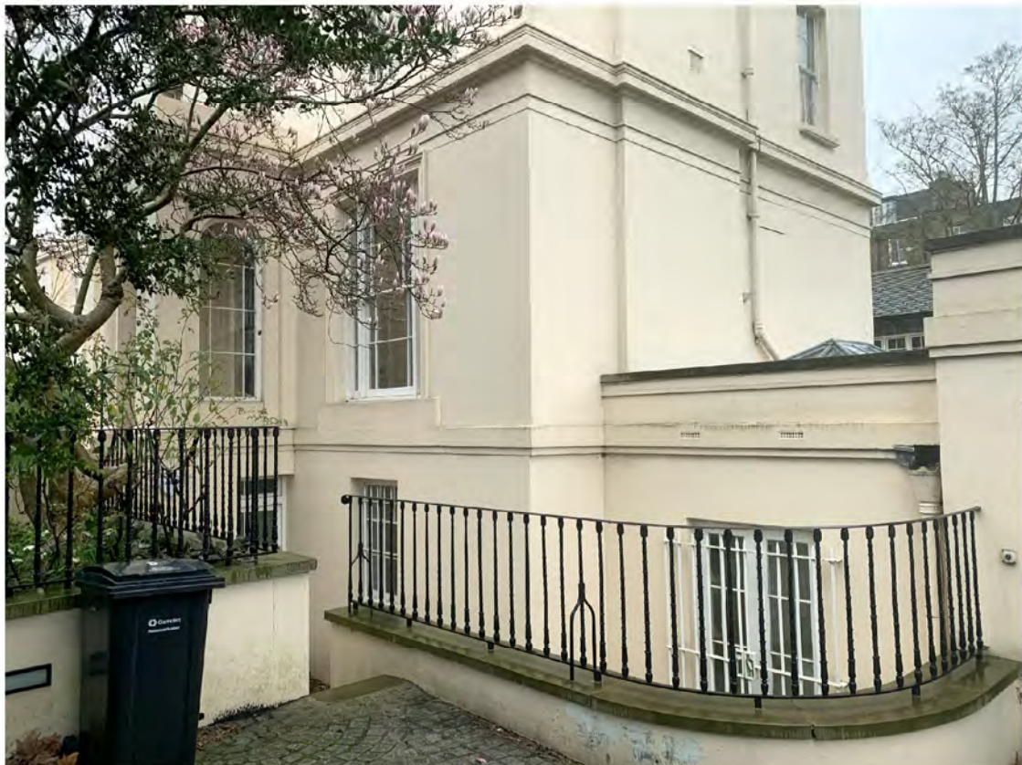
Plate 8: Railings to south and east elevations
