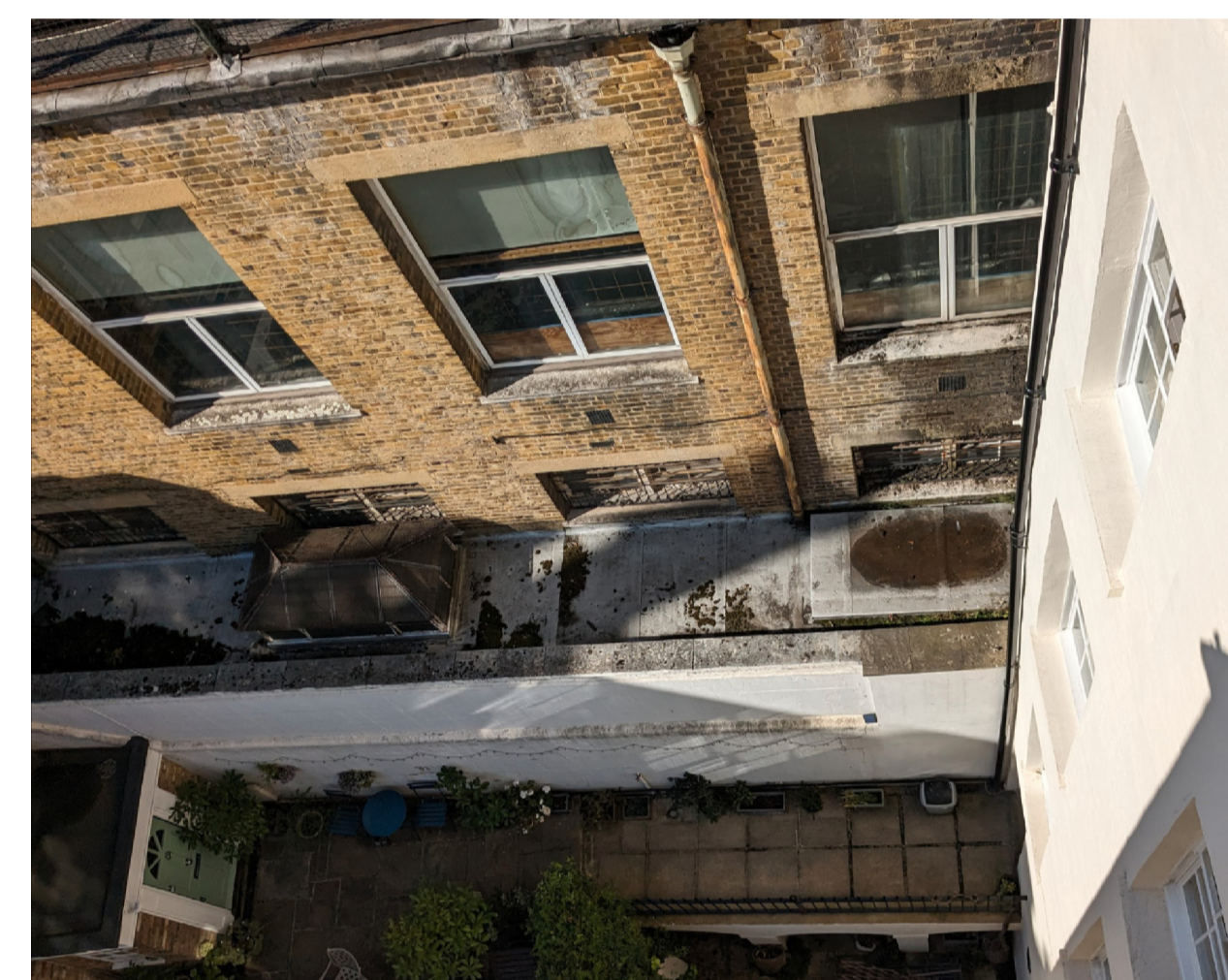
Photograph P2 From within 26 Old Gloucester Street showing Basement Level below.
