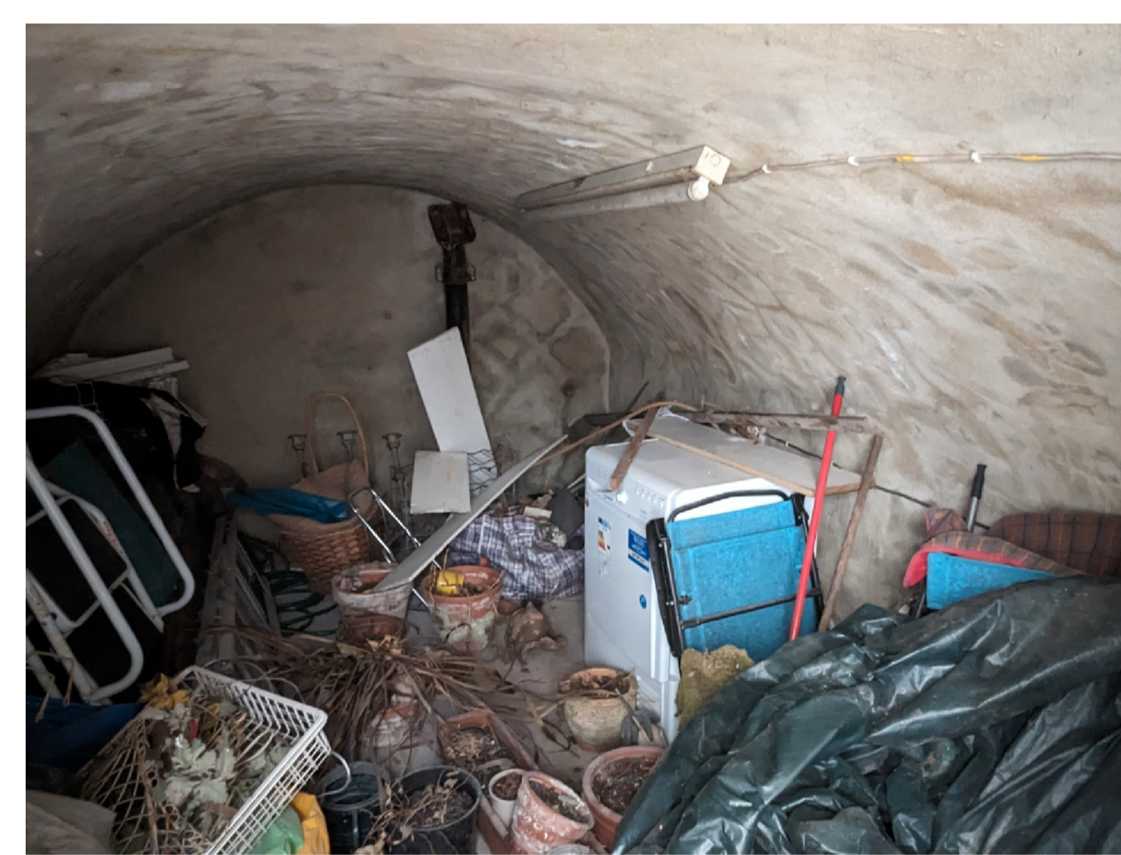
Photograph P3 From within 8 - 10 Cosmo Row at Basement Level.
