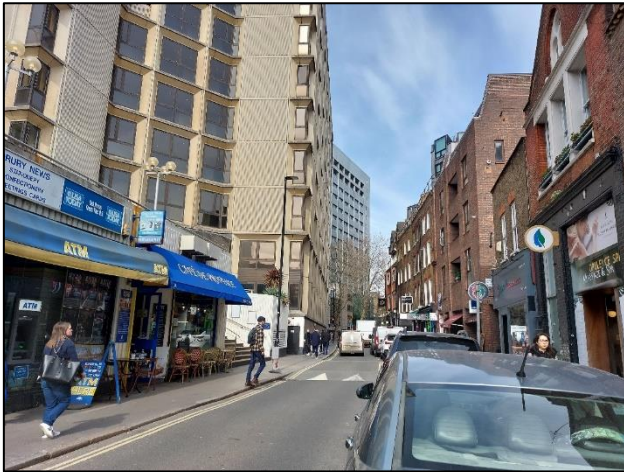
4.2 – View northwards up Drury Lane with the Site on the left and the asset within the terrace on the right.
