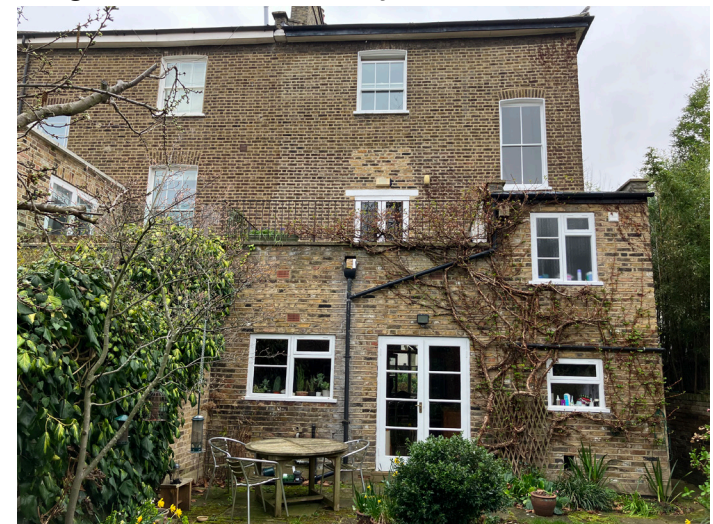
View of rear extension
