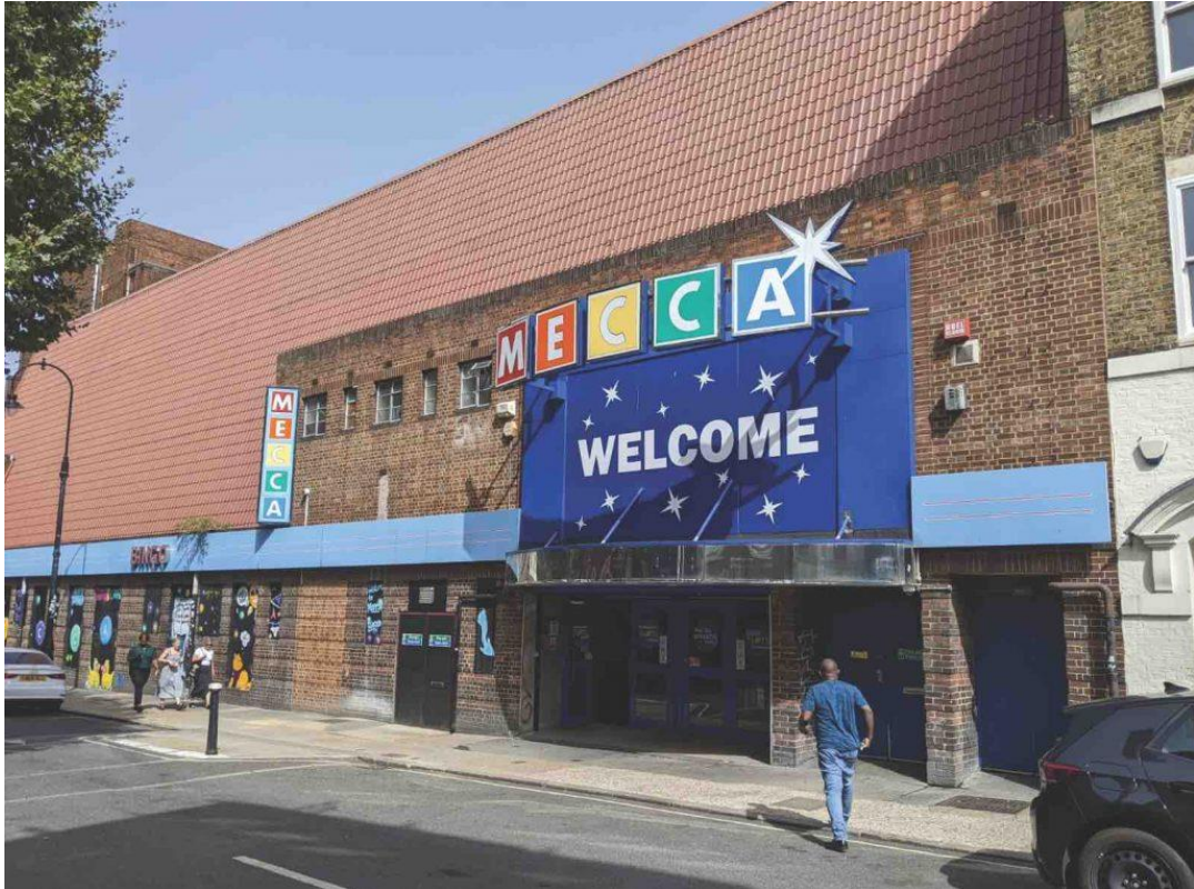
Figure 1 – The existing site
