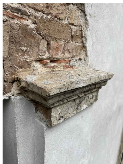
05 Plaster Capital as Existing 1000 NTS @ A3
