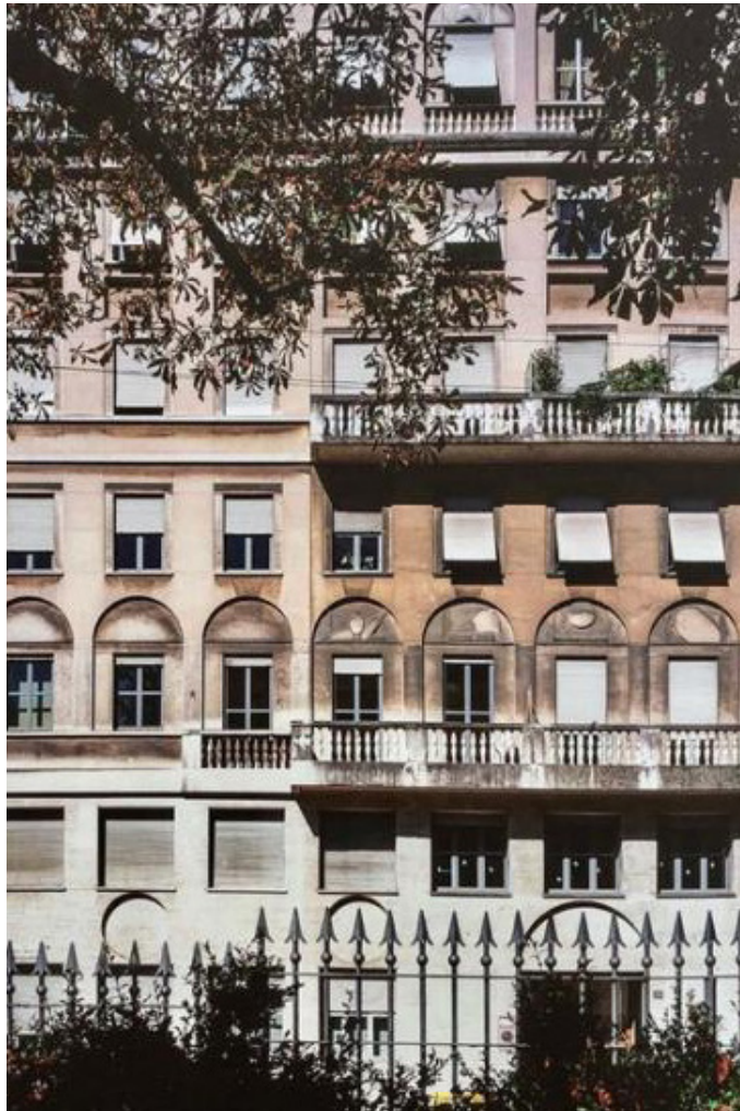
Facade with arched reveals and square window heads.
