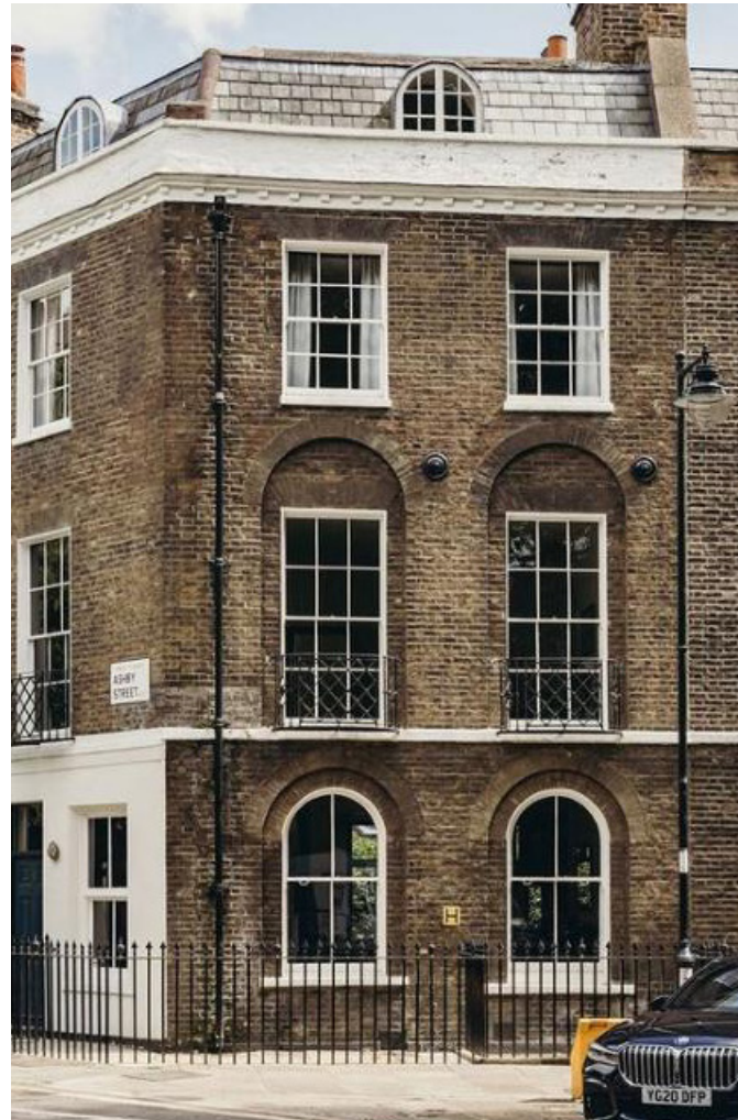
Georgian terrace of houses with varying windows. Brickwork and stucco detailing.
